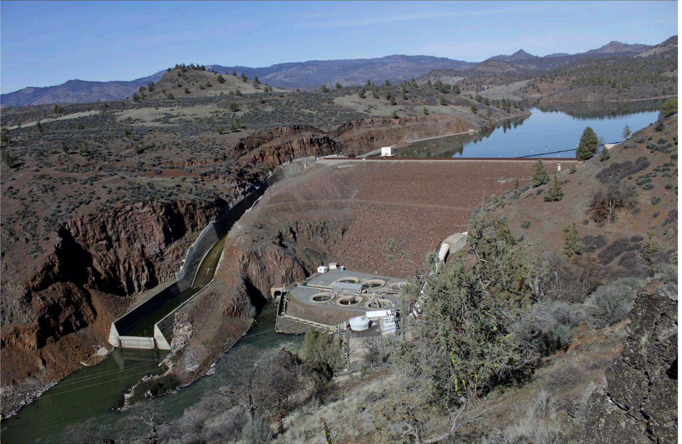
The Iron Gate Dam, powerhouse and spillway on the lower Klamath River near Hornbrook, Calif., Gillian Flaccus/Associated Press
