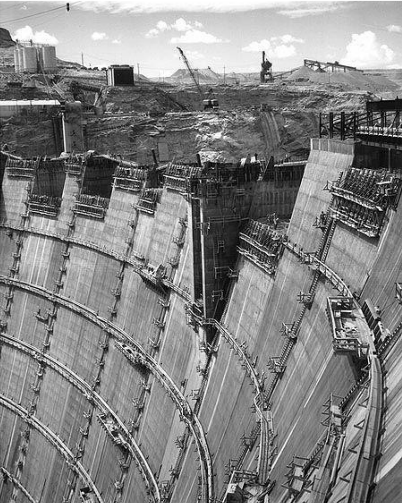
Construction of Glen Canyon Dam in 1963.
