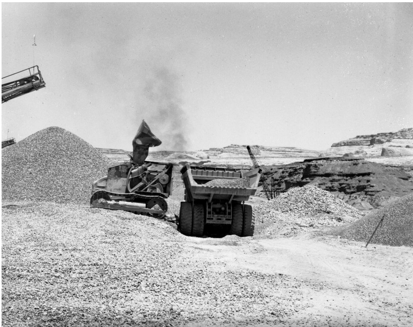
Heavy equipment moving rock at Glen Canyon Dam site, late 1950s.
