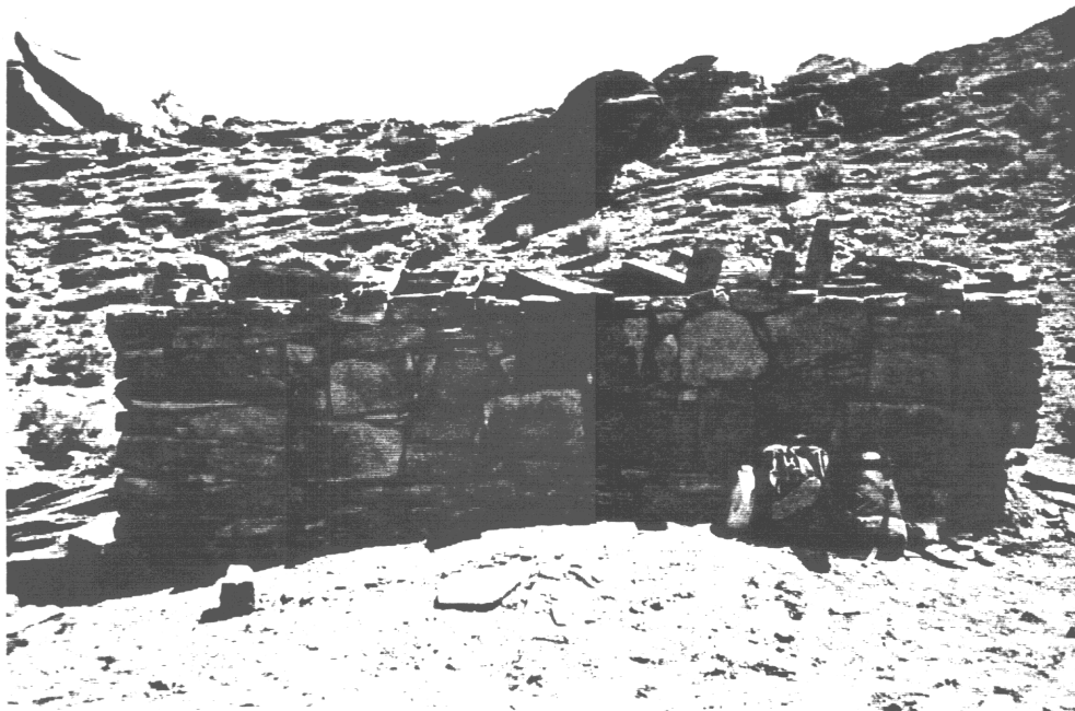
Figure 41. Vernacular sandstone structure opposite Lees Ferry (NPS project photo 1991).
