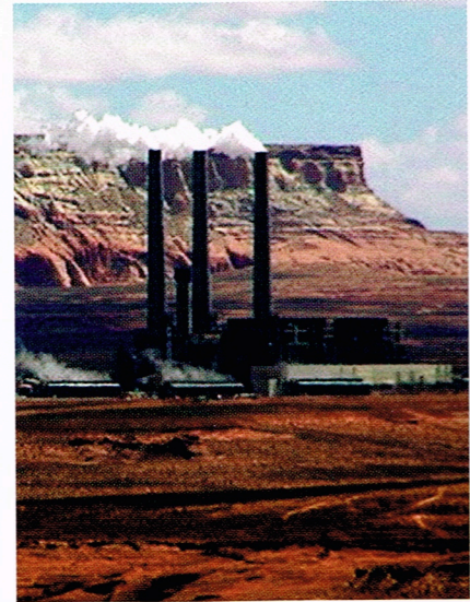
Navajo Power Plant
