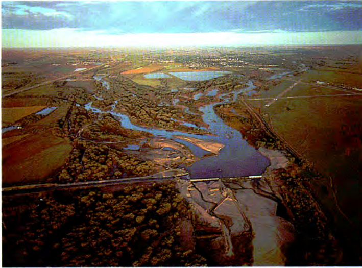
Keystone Dam on the Platte River
