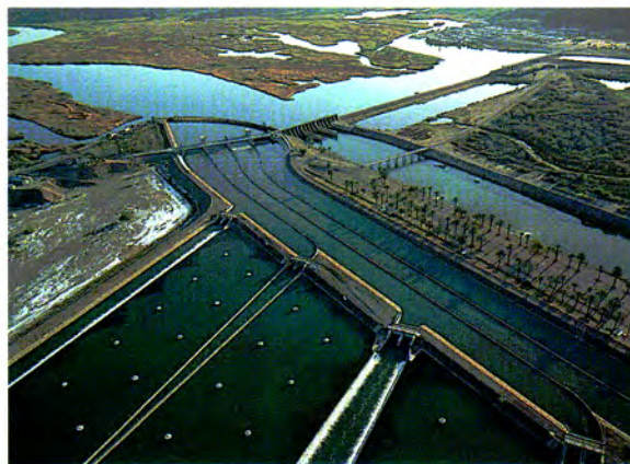
Imperial Dam north of Yuma Arizona
