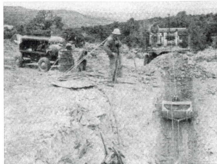
Slushing operation at the Yellow Circle Mine.
