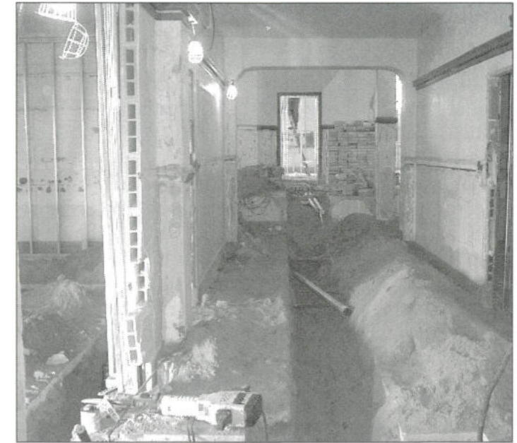
The photographs on this page were taken by Layton Construction during the renovation process. They show the geothermal wells being dug on the property, and the pipes that help move the temperatures of the earth into the buildings.
