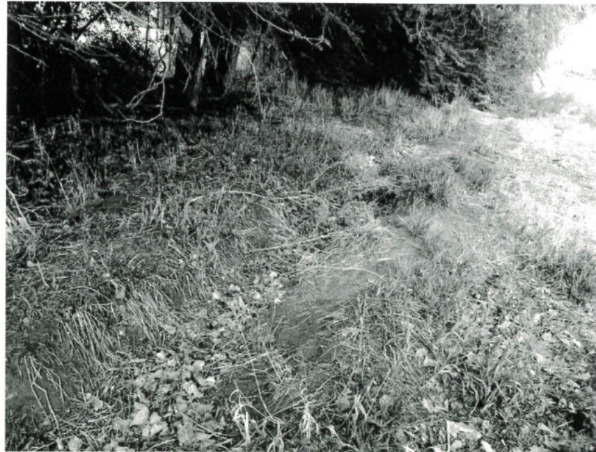
The remains of the irrigation ditch dug by the missionaries to bring water from nearby springs to their fields. The ditch was nearly one mile in length.
