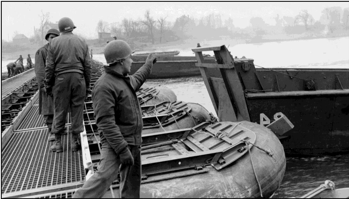
Section of Army Treadway bridge being pushed into place by LCV on Rhine River near Remagen Bridge
