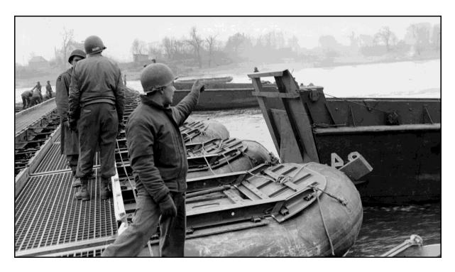
Section of Army Treadway bridge being pushed into place by LCVP on Rhine River near Remagen Bridge
