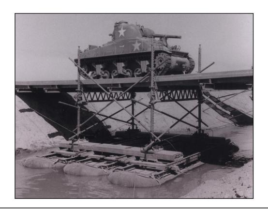
Above: Sherman M-4 Tank crossing a unique pontoon bridge at Yuma Testing Ground.
