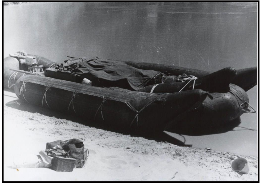
{ARTA - 33' Pontoon w 2 outrigger tubes outside & one inside}
