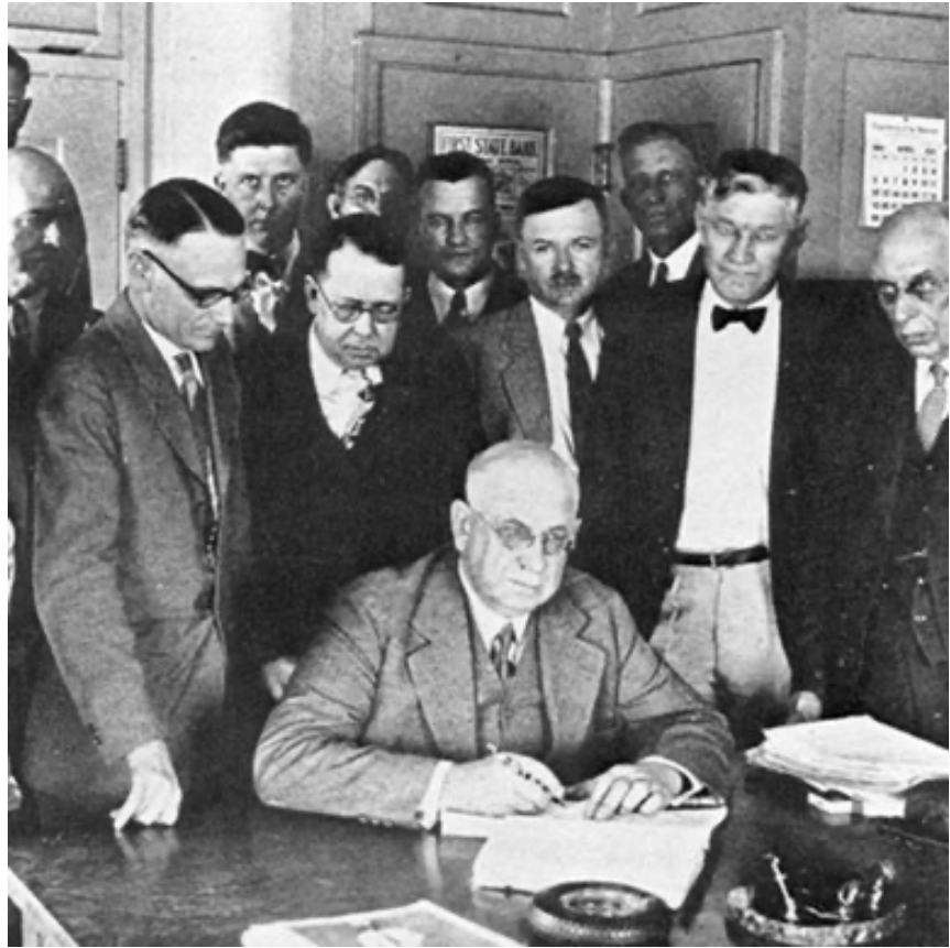
Reclamation signs contract to begin Hoover Dam construction
