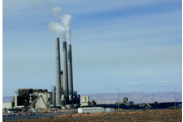
Navajo Generating Station, Page AZ
