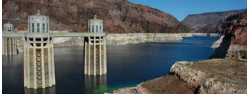
Intake towers at Hoover Dam
