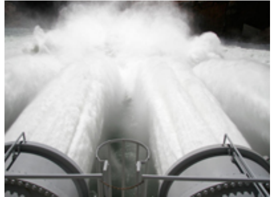
Jet tubes at Glen Canyon Dam mimic natural floods
