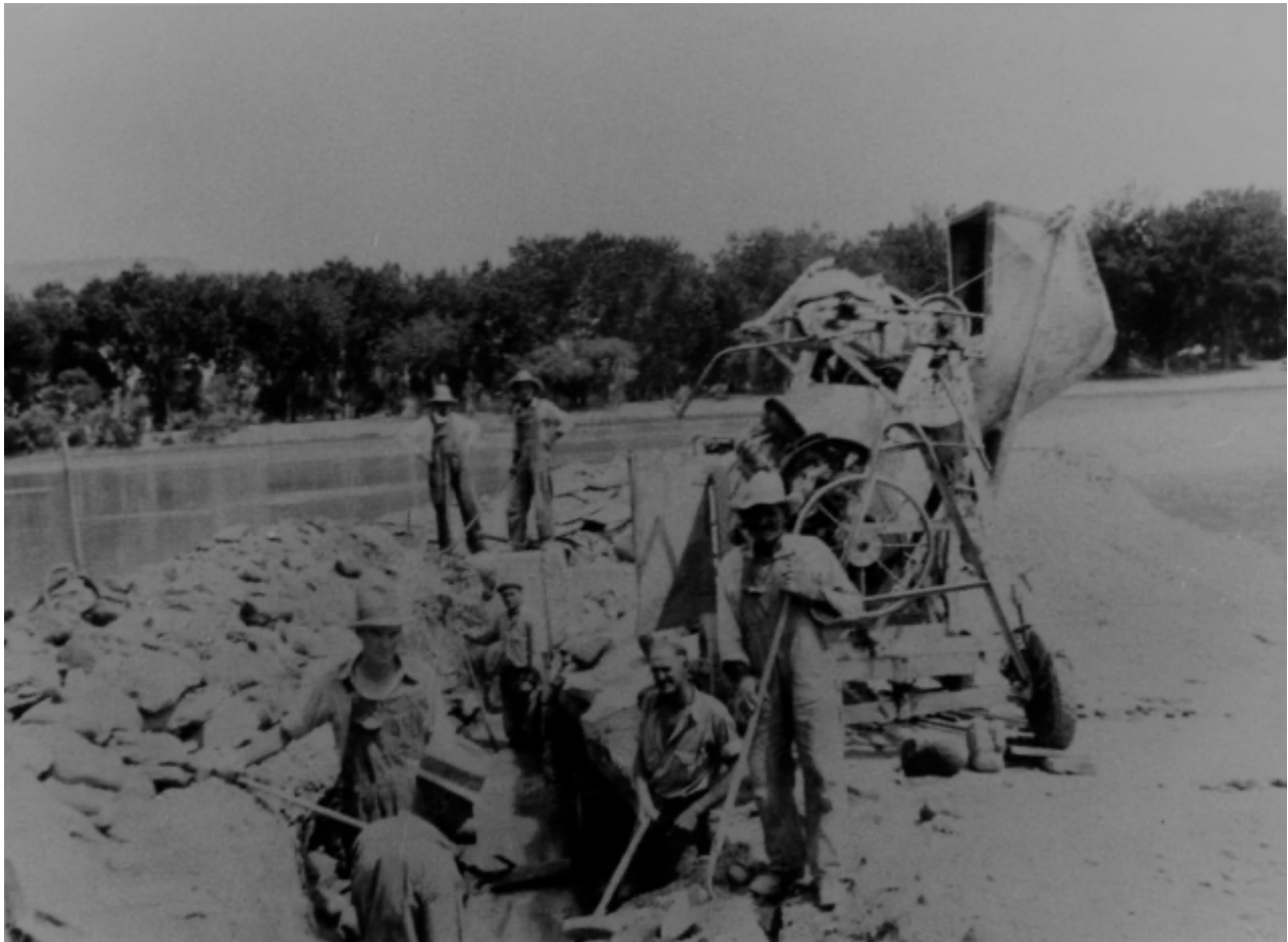
Tusher Wash Dam construction in 1936
