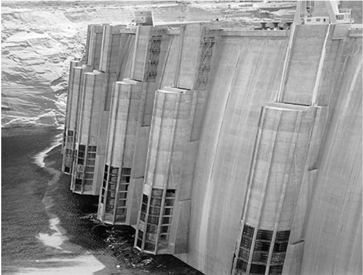
Glen Canyon Dam during initial filling in 1963
