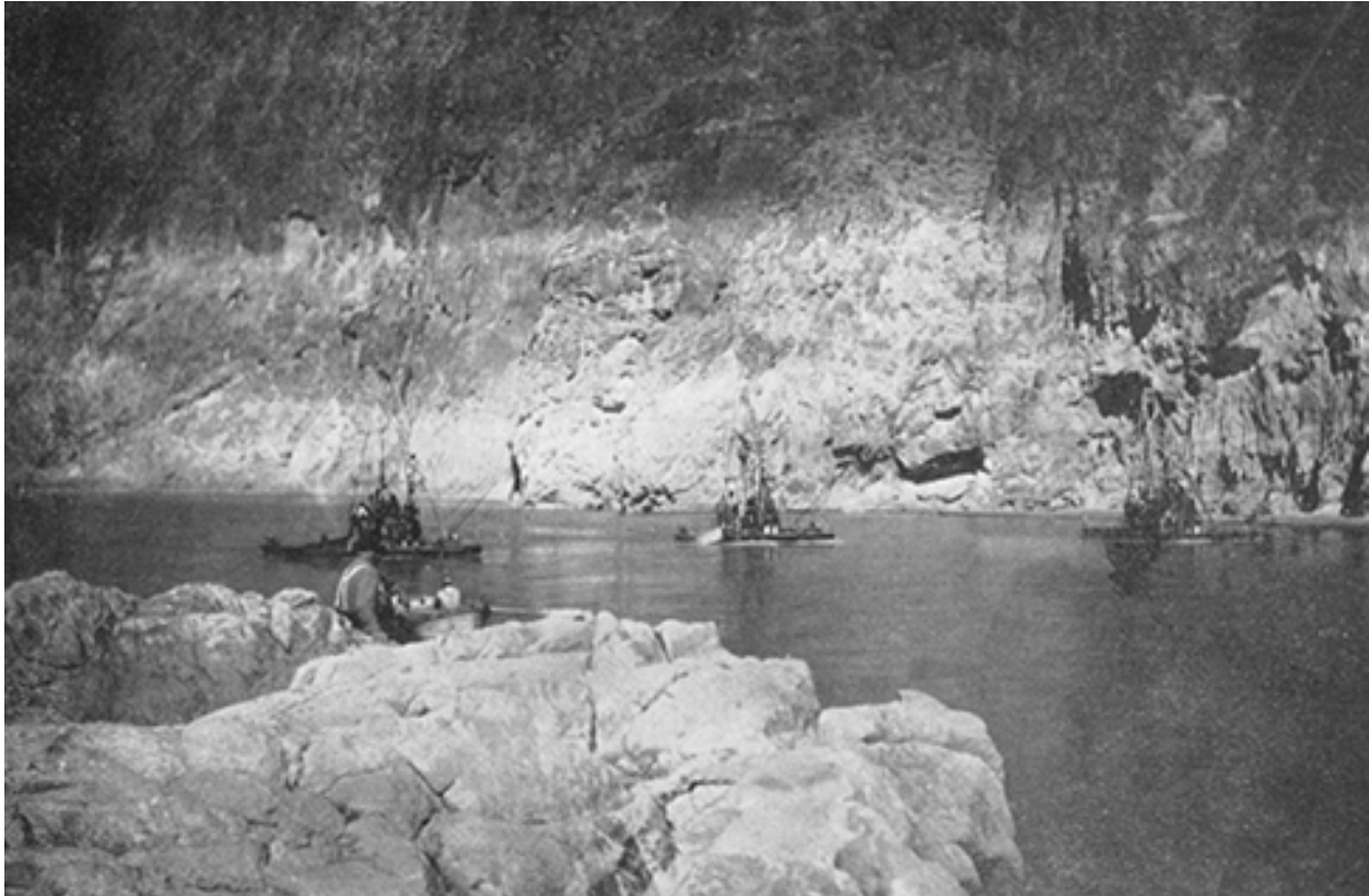
USGS photo, circa 1925. Drilling crew examining bedrock at constricted Boulder Canyon. Note high water scour line 80 feet above low water level.
