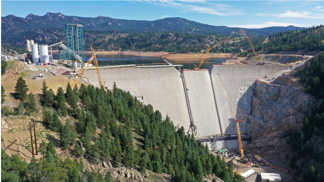
The construction site of the Gross Reservoir Dam expansion in 2024. Credit: Denver Water
