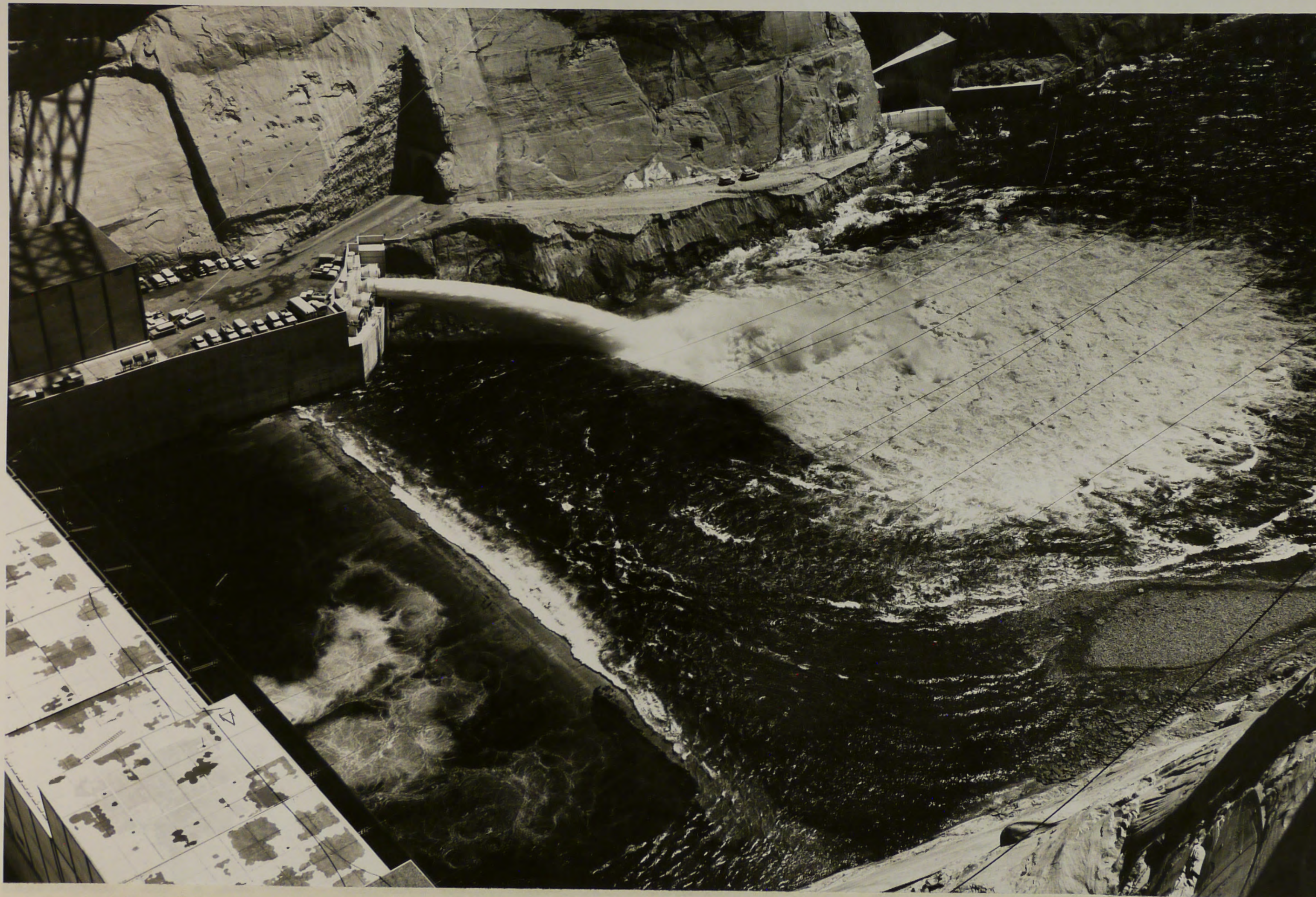
P 557-420-10855 Glen Canyon Unit--C.R.S.P. NA Flow through Outlet Gate No. 3, showing eddying at tailrace slab.
