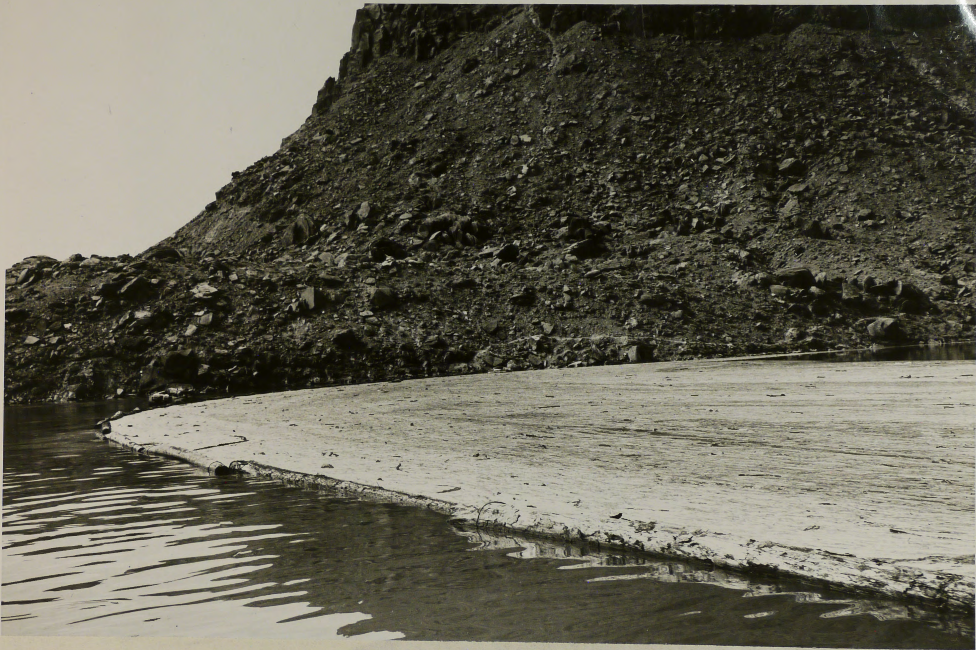
P 557-420-10902- Glen Canyon Unit--C.R.S.P. NA Log barrier constructed across San Juan River preventing oil flow into Lake Powell. 4-21-65
