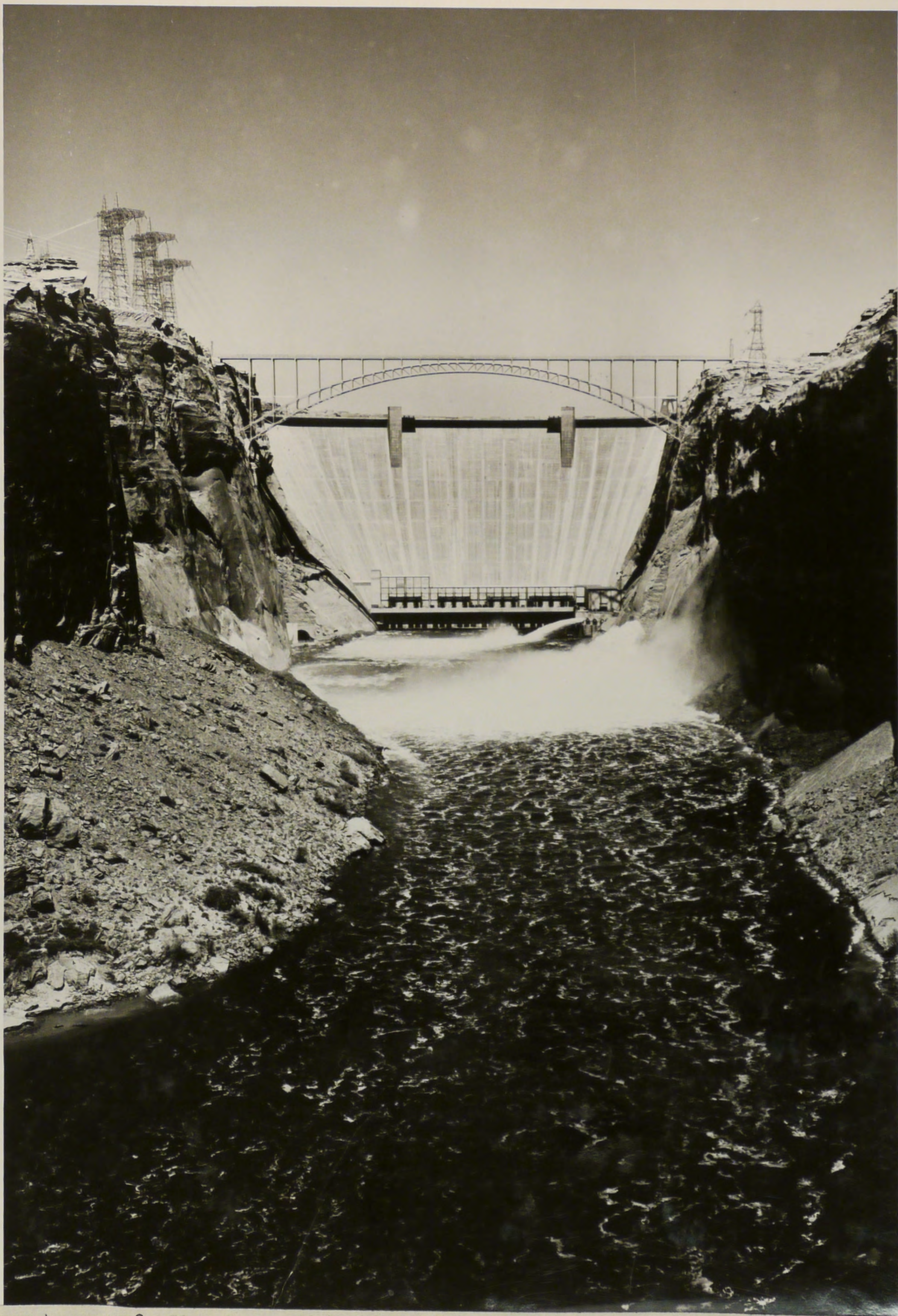
P 557-420-10918 Glen Canyon Unit--C.R.S.P. NA View of tailrace area showing discharge from Outlet Gate No. 1 and left diversion tunnel. 4-29-65 F. Finch
