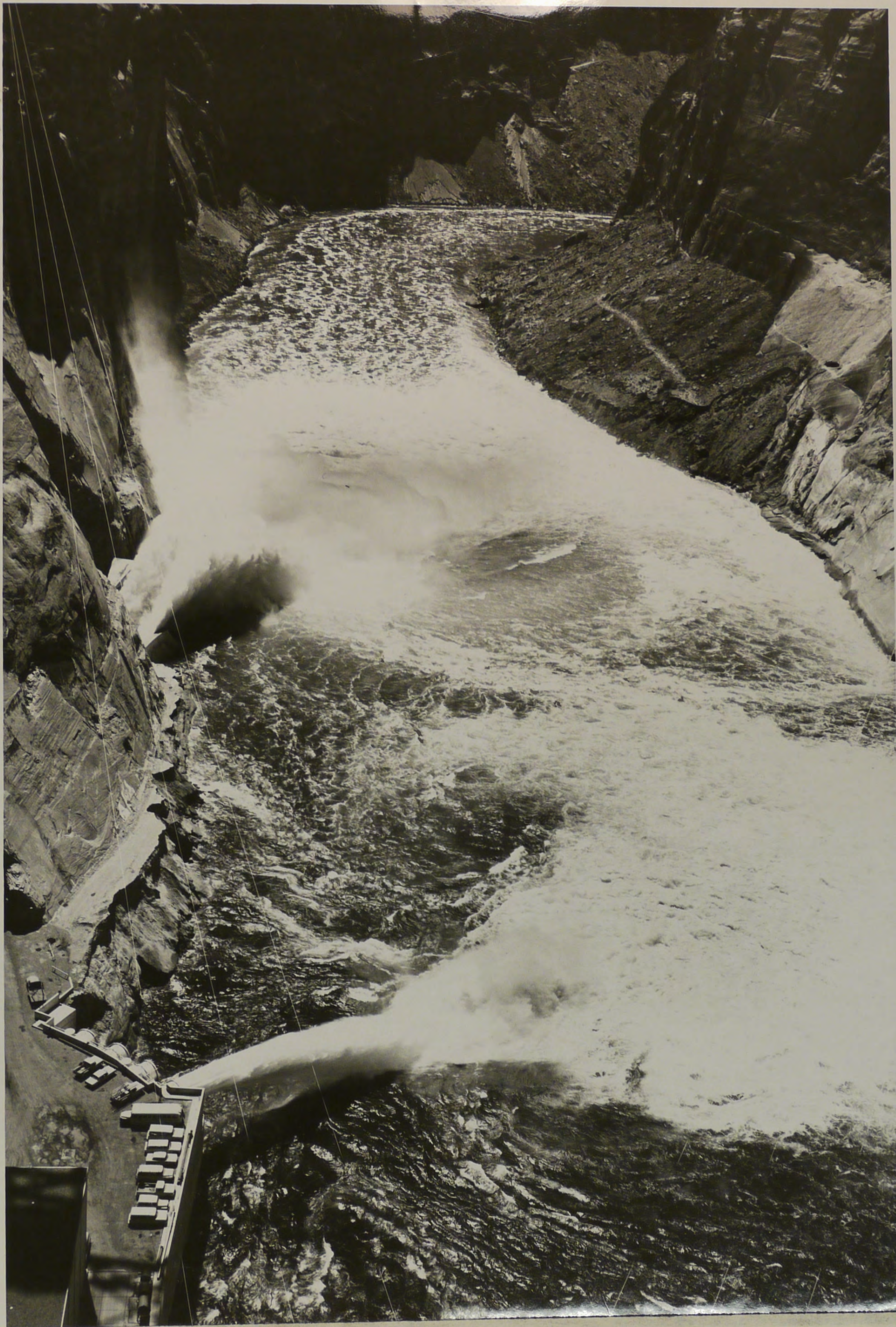
P 557-420-10916 Glen Canyon Unit--C.R.S.P. NA Looking downstream from power plant. No. 1 river outlet and left flip bucket in operation. 4-29-65 F. Finch
