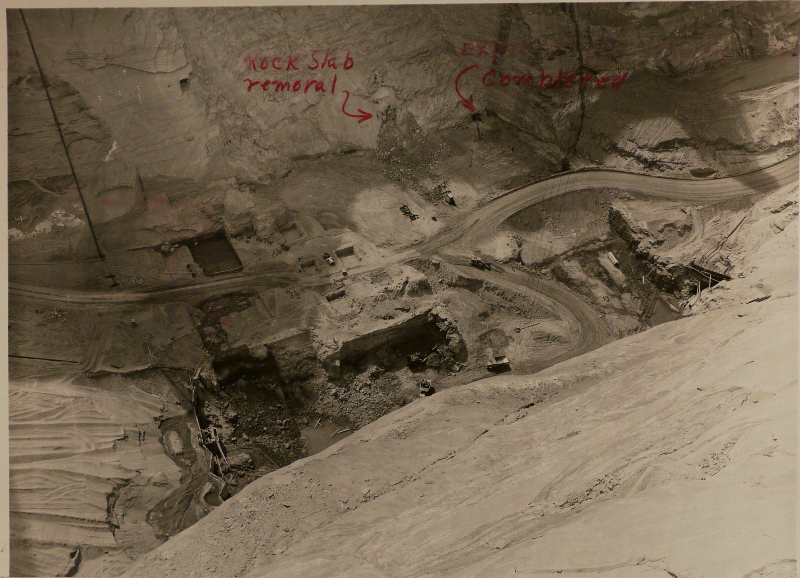
P 557-420-04731 Glen Canyon Unit--C.R.S.P. Power plant excavation and base of right keyway. Five penstock support footing excavation sites in center. Contractor: Merritt-Chapman and Scott Corporation, Contract No. 14-06-D-2403. Specs. No. DC-4825. 4-21-60 A. E. Turner
