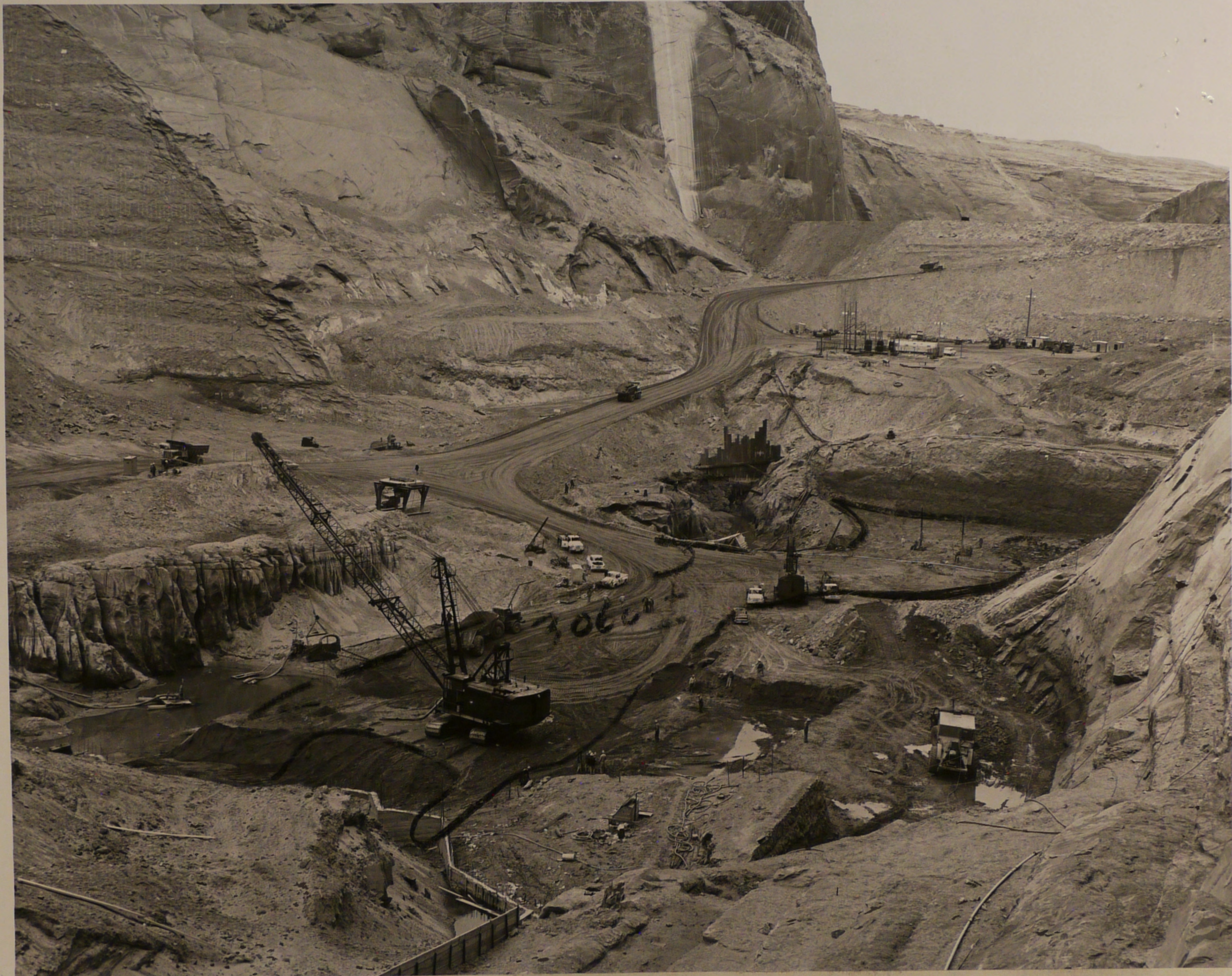
P 557-420-04475 Glen Canyon Unit--C.R.S.P. Looking upstream at operations in the river bottom for the power plant structure site and the dam foundation. Contractor: Merritt-Chapman and Scott Corporation, Contract No. 14-06-D-2403. Specs. No. DC-4825. 3-3-60 A. E. Turner
