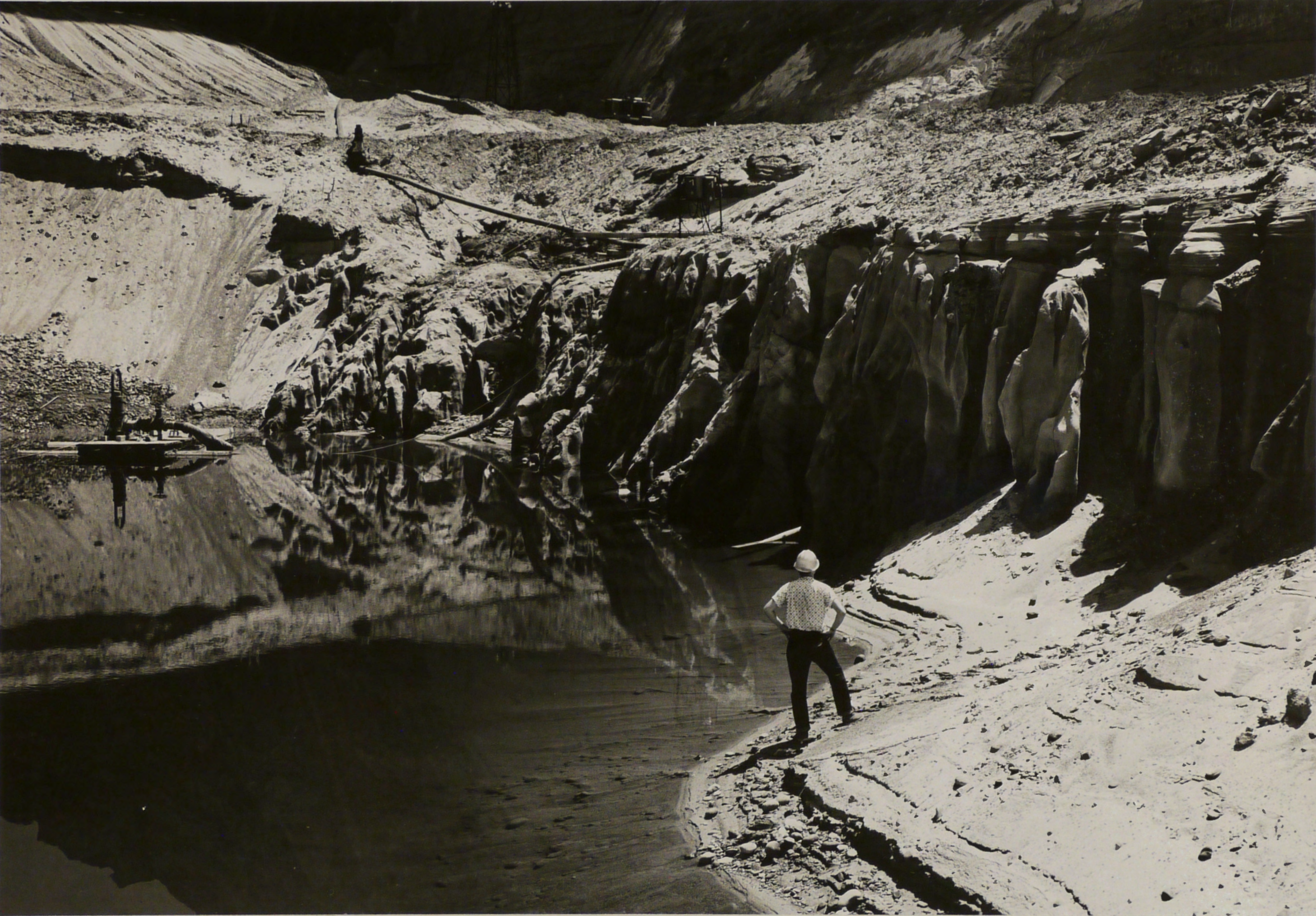
P 557-420-04017 Glen Canyon Unit--Colorado River Storage Project. Excavation for the dam foundation in the river bottom showing eroded rock. Contractor: Merritt- Chapman and Sockt Corporation, Contract No. 14-06-D-2403. Specs. No. DC-5825. 7-17-59
