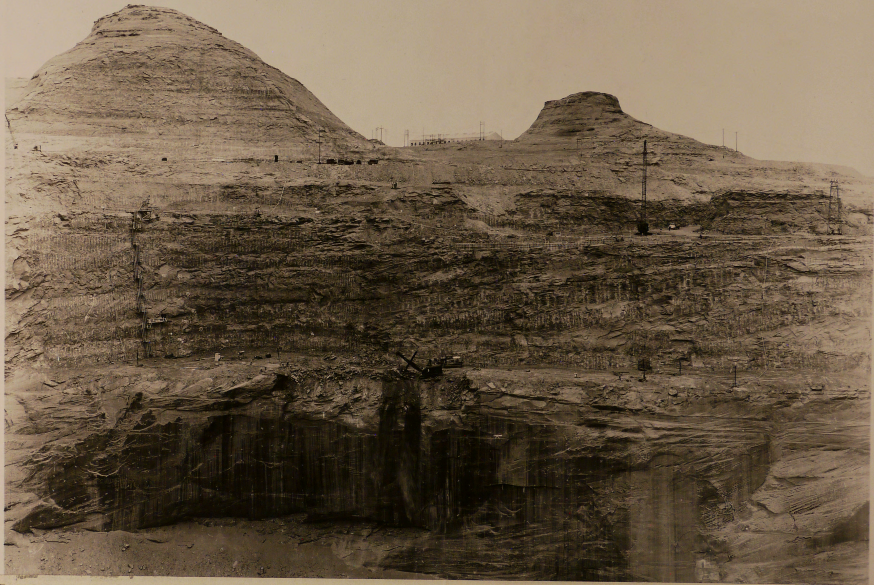
P 557-420-2330 Glen Canyon Unit--Colorado River Storage Project. Excavation in right keyway of the dam showing ladders for access to the work. Foundation tunnel can be seen at right of platform extending to right of ladders. Contractor: Merritt-Chapman and Scott Corporation, Contract No. 14-06-D-2403. Specs. No. DC-4825. A. E. Turner
