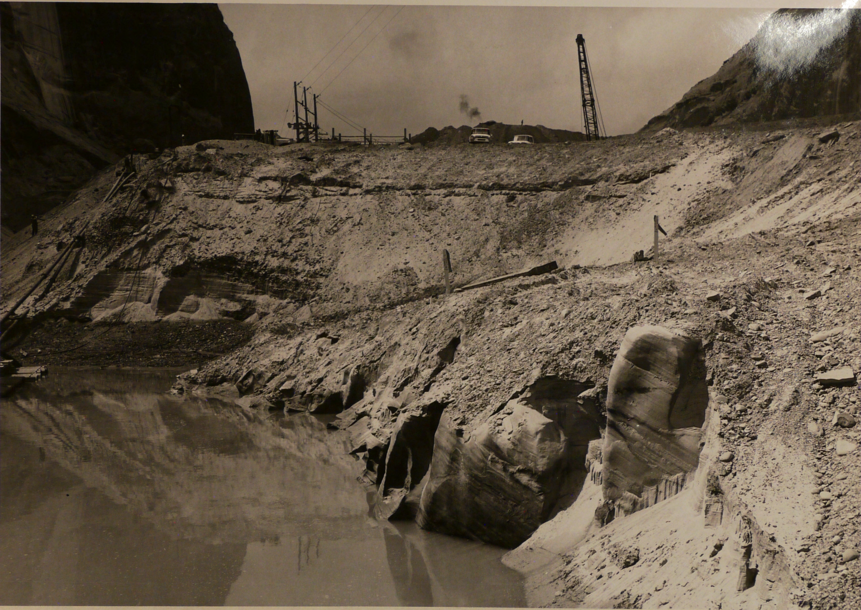
P 557-420-03843 Glen Canyon Unit--Colorado River Storage Project. Pot holes and flutes in the sandstone uncovered along the left side of the dam foundation excavation. Contractor: Merritt-Chapman & Scott Corporation, Contract No. 14-06-D-2403. Specs. No. DC-4825. 5-29-59 A. E. Turner
