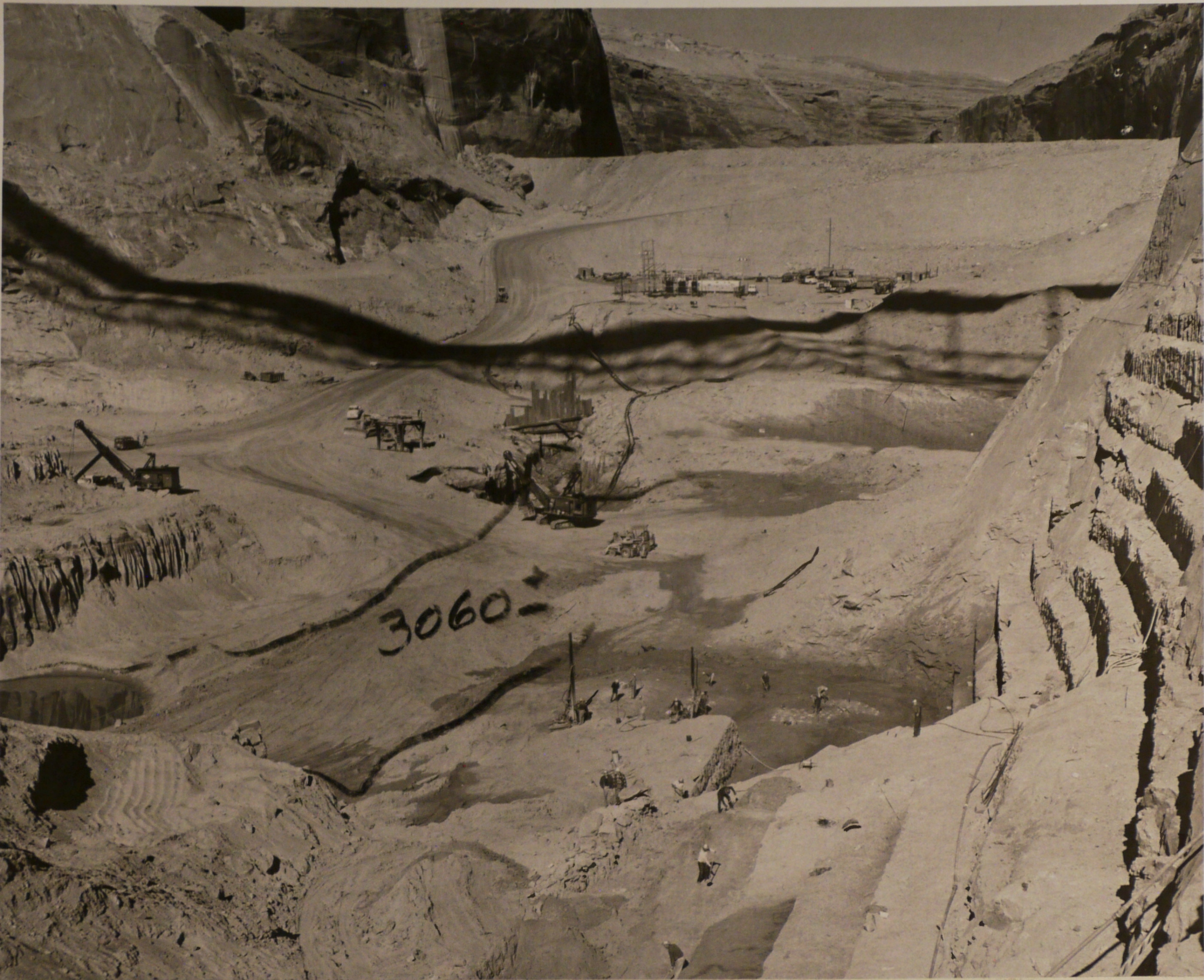
P 557-420-04361 Glen Canyon Unit--C.R.S.P. Progress of excavation for the dam foundation in the river bottom. Contractor: Merritt-Chapman and Scott Corporation, Contract No. 14-06-D-2403. Specs. No. DC-4825. 2-4-60 A. E. Turner
