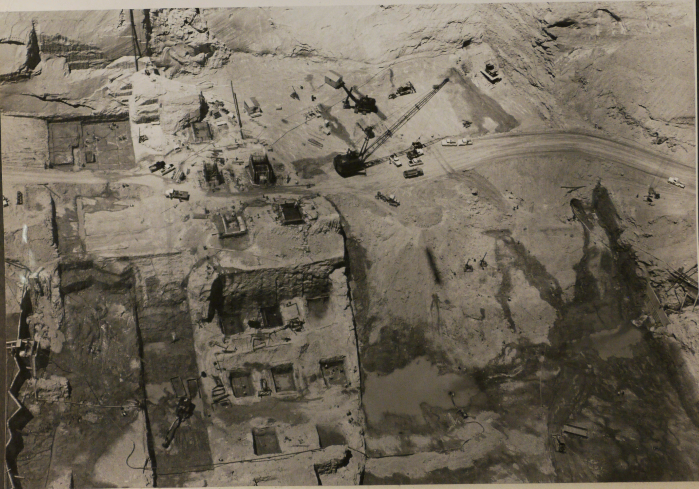
P 557-420-04838 Glen Canyon Unit--C.R.S.P. Looking down at the excavation area in the river bottom and on the right side of the canyon. Penstock support footings through left center. Excavation for ground mat in Unit Bays 1 and 3. Contractor: Merritt-Chapman and Scott Corporation, Contract No. 14-06-D-2403. Specs. No. DC-4825. 5-19-70 A. E. Turner
