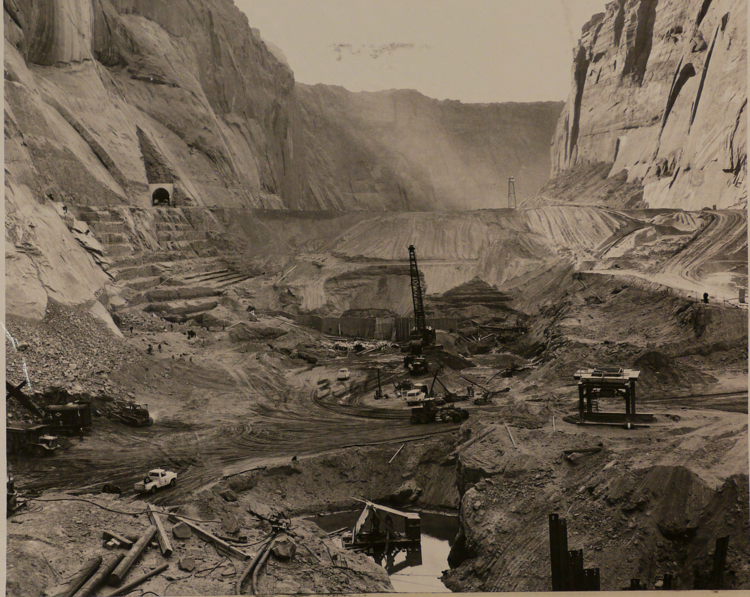
P 557-420-04441 Glen Canyon Unit--C.R.S.P. Progress of excavation in the river bottom for the dam foundation. Contractor: Merritt-Chapman and Scott Corporation, Contract No. 14-06-D-2403. Specs. No. DC-4825. 2-25-60 A. E. Turner
