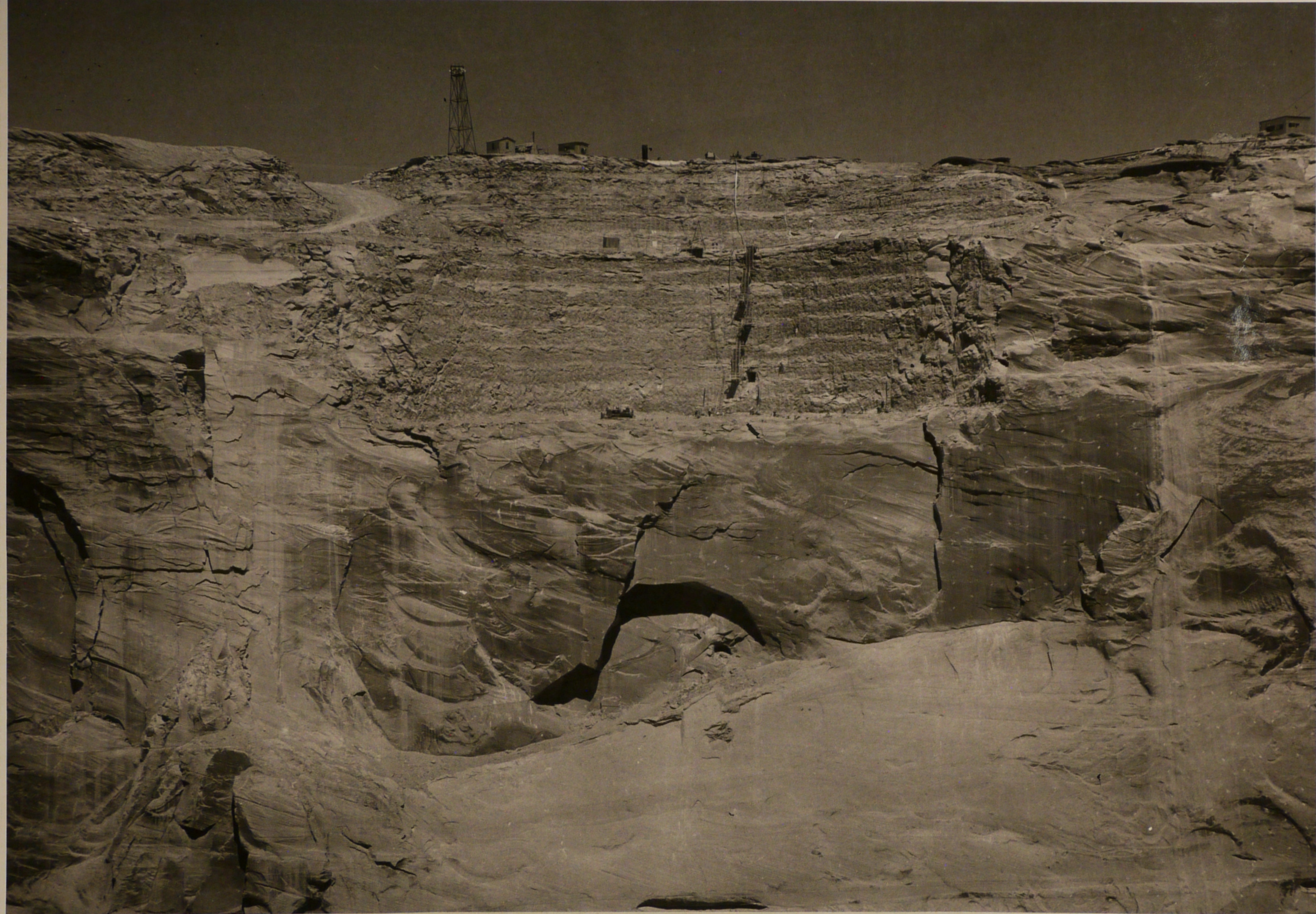
P 557-420-2307 Glen Canyon Unit--Colorado River Storage Project. Left keyway of the dam. Left foundation tunnel can be seen near lower platform of ladder sections. Contractor: Merritt-Chapman and Scott Corporation, Contract No. 14-06-D-2403. Specs. No. DC-4825. 6/2/58 A. E. Turner
