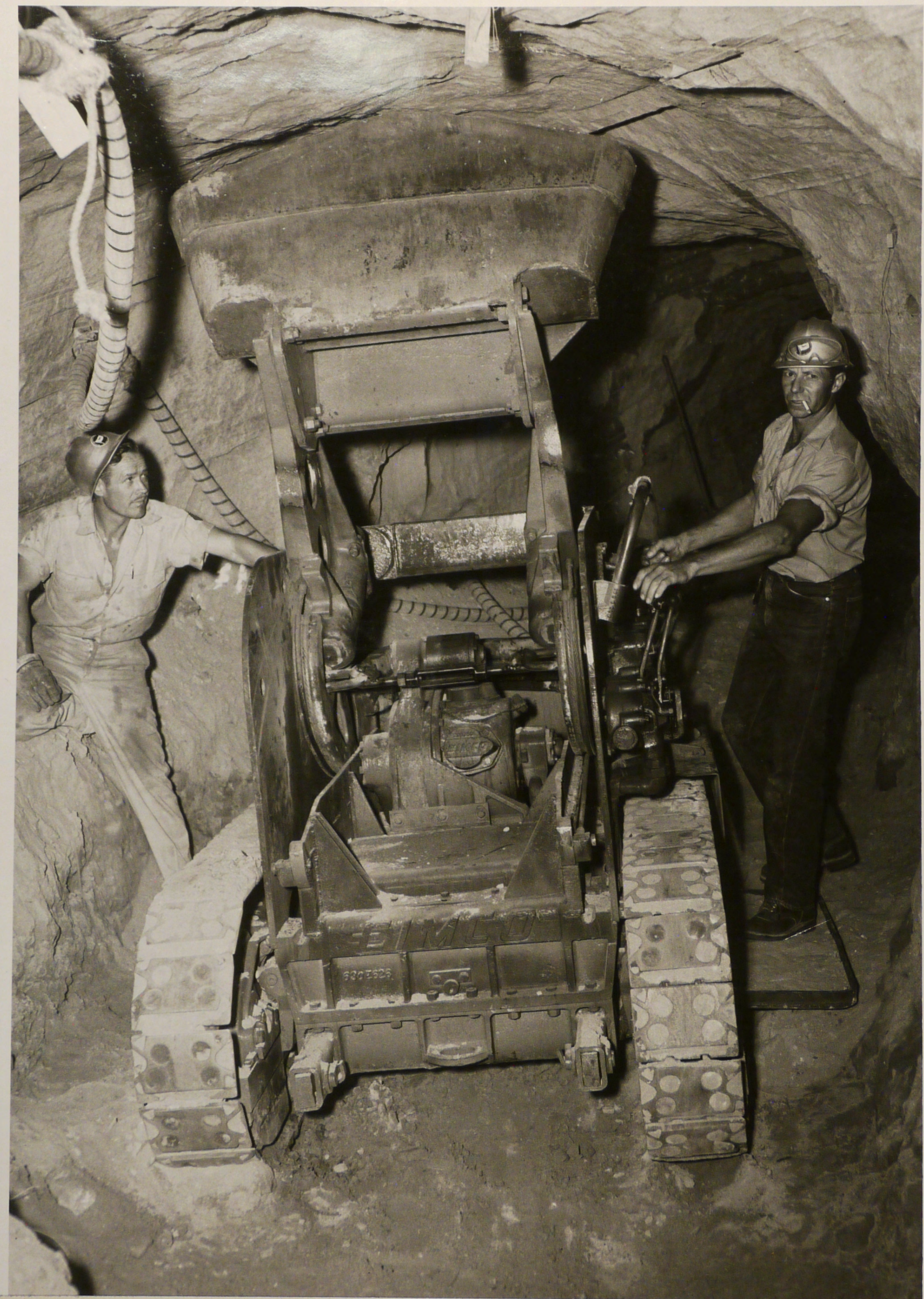
P 557-420-2297 Glen Canyon Unit--Colorado River Storage Project. Workmen of Merritt-Chapman and Scott Corporation operate Eimco loader in the right foundation tunnel. Contract No. 14-06-D-2403; Specs. No. DC-4825. 6/2/58 A. E. Turner
