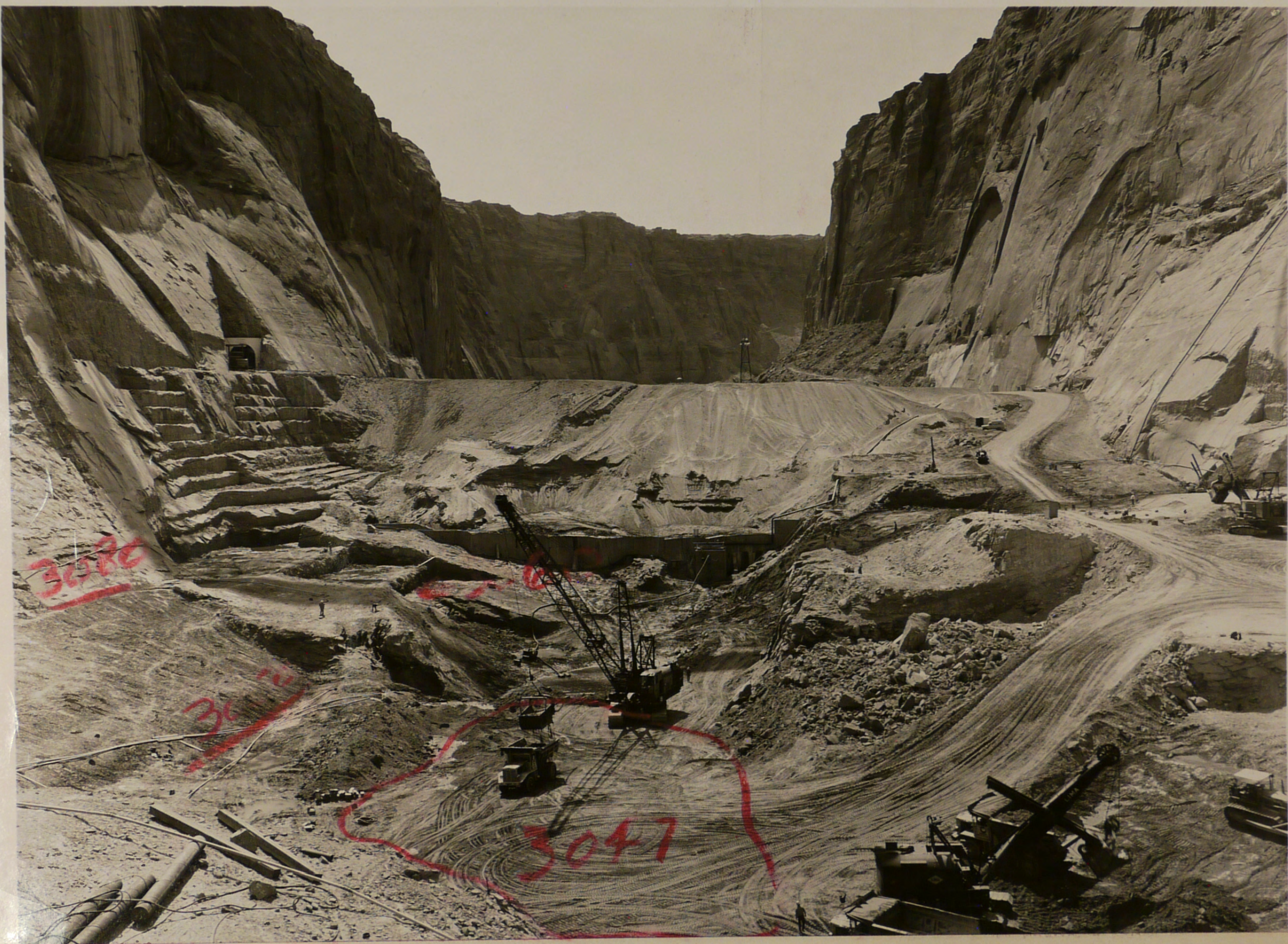
P 557-420-04642 Glen Canyon Unit--C.R.S.P. Looking downstream at excavation for the dam foundation and for the power plant in the river bottom. Contractor: Merritt-Chapman and Scott Corporation, Contract No. 14-06-D-2403. Specs. No. DC-4825. 4-7-60 A. E. Turner
