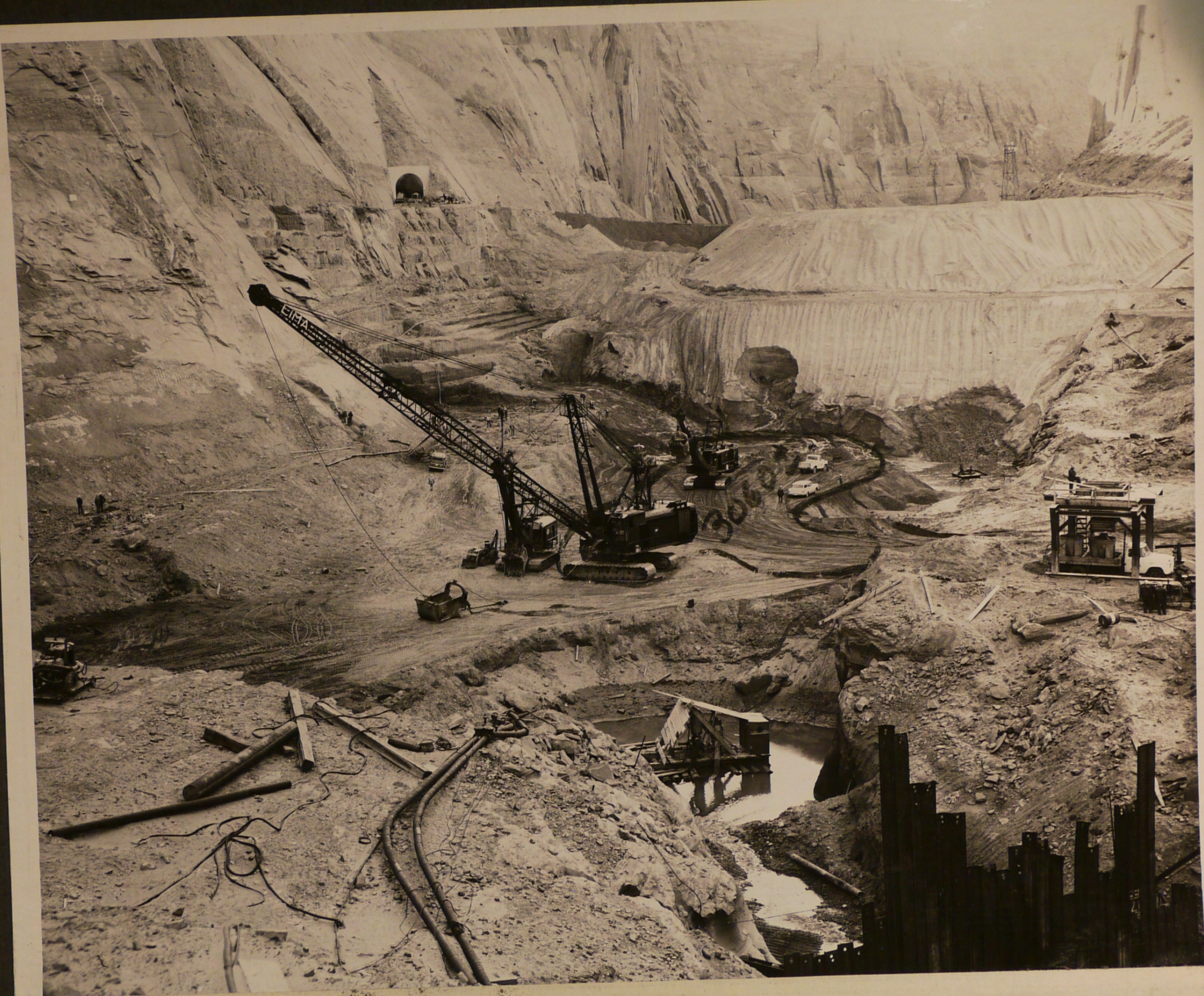
P 557-420-04382 Glen Canyon Unit--G.R.S.P. Looking downstream in the river bottom area. Note water seeping through downstream coffer- dam to sump. Contractor: Merritt-Chapman and Scott Corporation, Contract No. 14-06-D-2403. Specs. No. DC-4825. 2-11-60 A. E. Turner
