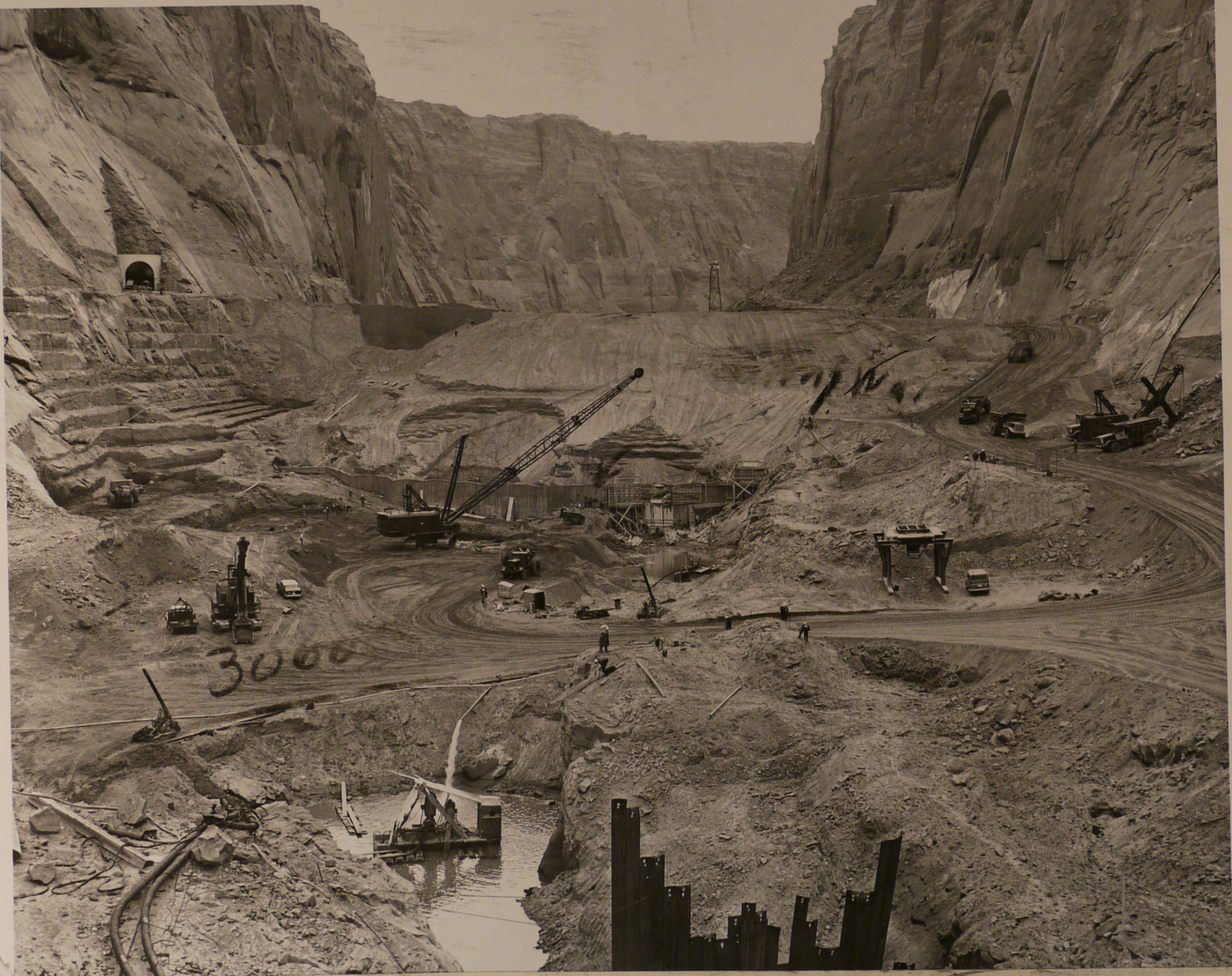
P 557-420-04474 Glen Canyon Unit--C.R.S.P. Looking downstream at progress of operations in the river bottom. Contractor: Merritt-Chapman and Scott Corporation, Contract No. 14-06-D-2403. Specs. No. DC-4825. 3-3-60 A. E. Turner
