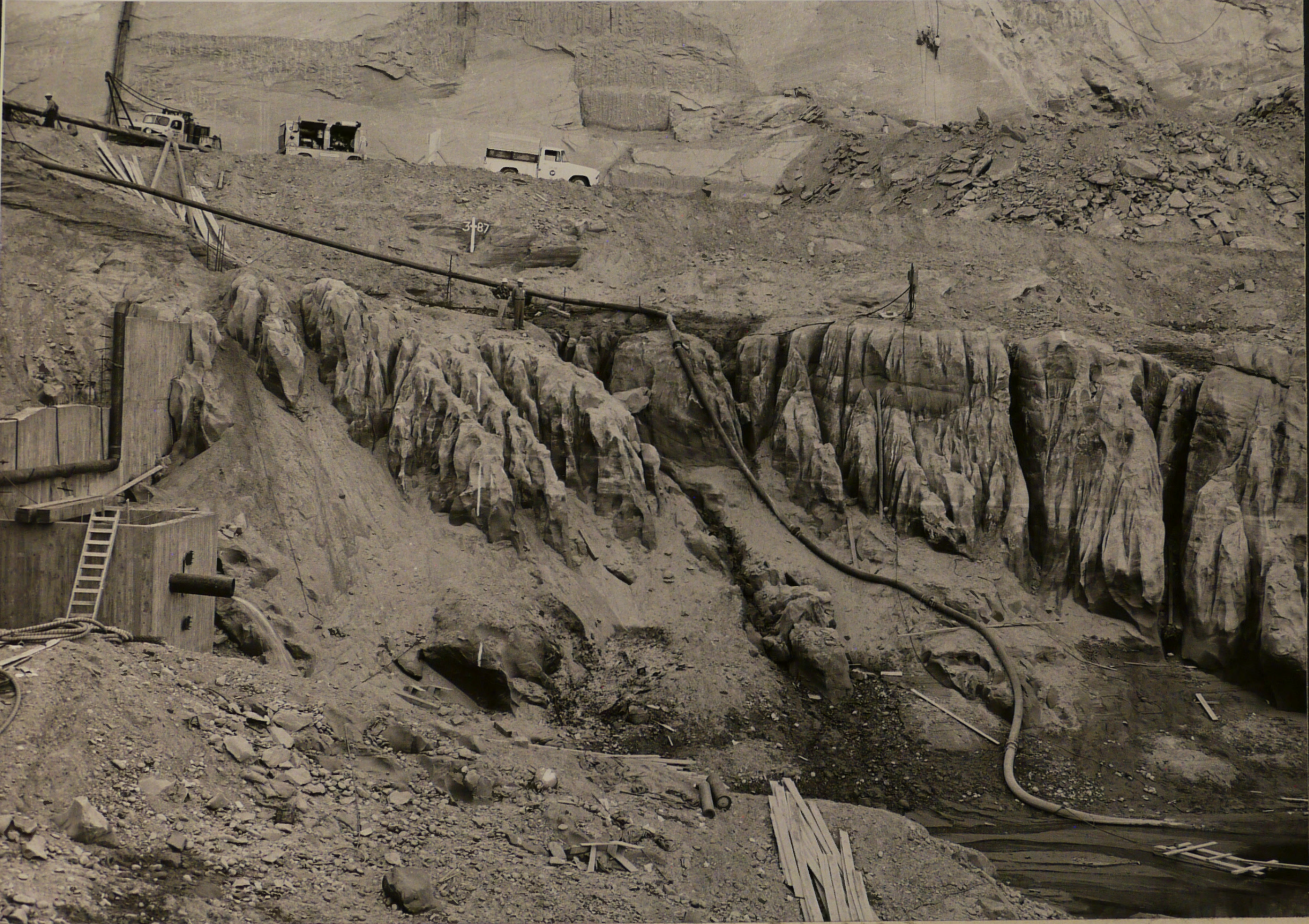
P 557-420-04536 Glen Canyon Unit--C.R.S.P. Contractor's concrete sump and excavation for power plant structure in the inner gorge. Contractor: Merritt-Chapman and Scott Corporation, Contract No. 14-06-D-2403, Specs. No. DC-4825. 3-22-60 A. E. Turner
