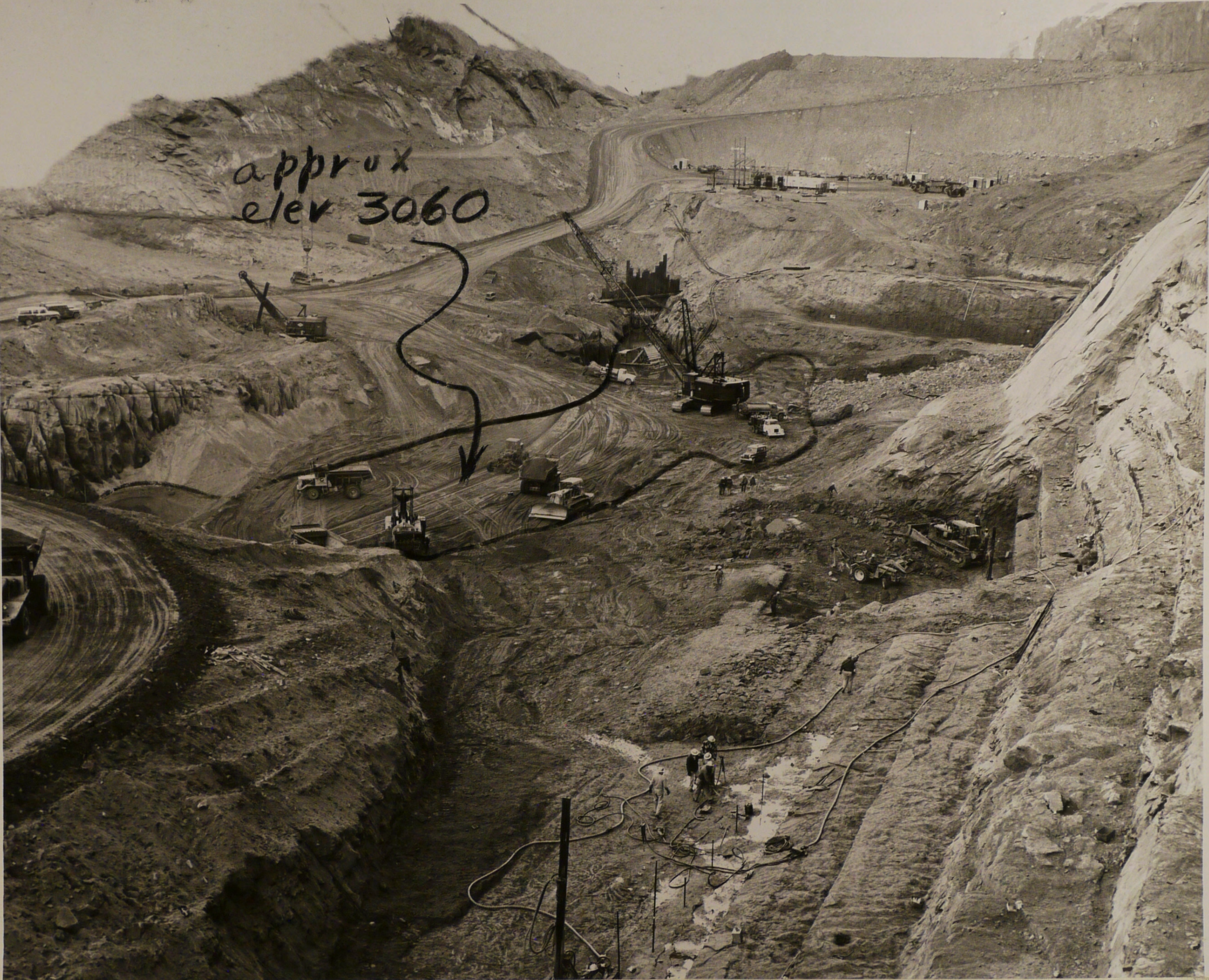
557-420-04326 Glen Canyon Unit--C.R.S.P. Progress of excavation for the dam foundation in the river bottom. Contractor: Merritt-Chapman and Scott Corporation, Contract No. 14-06-D-2403. Specs. No. DC-4825. 1-28-60 A. E. Turner
