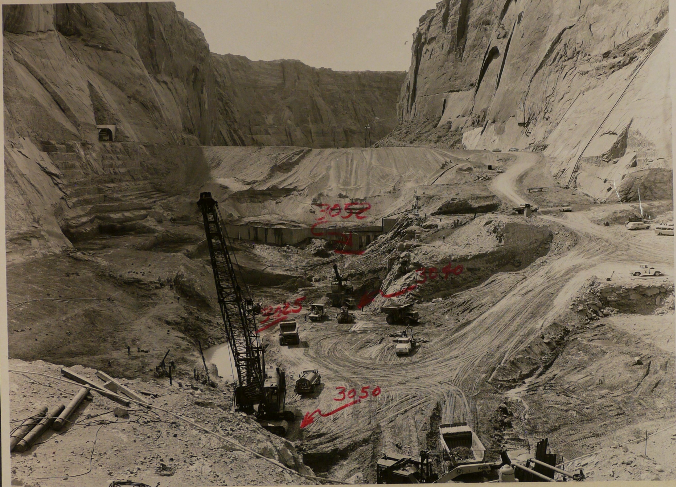
P 557-420-04683 Glen Canyon Unit--C.R.S.P. Looking downstream at dam foundation and powerplant structure excavation. Contractor: Merritt-Chapman and Scott Corporation. Contract No. 14-06-D-2403. Specs. No. DC-4825. 1. 11. 60 A. E. Turner
