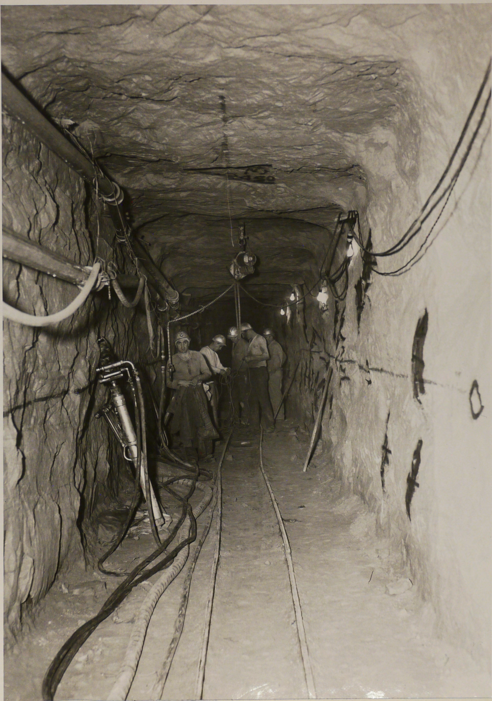
557-420-03251 Glen Canyon Unit--Colorado River Storage Project. Right foundation tunnel at elevation 3,247 \pm . Contractor: Merritt- Chapman & Scott Corporation, Contract No. 14-06-D-2403. Specs. No. DC-4825. 1/22/59 A. E. Turner
