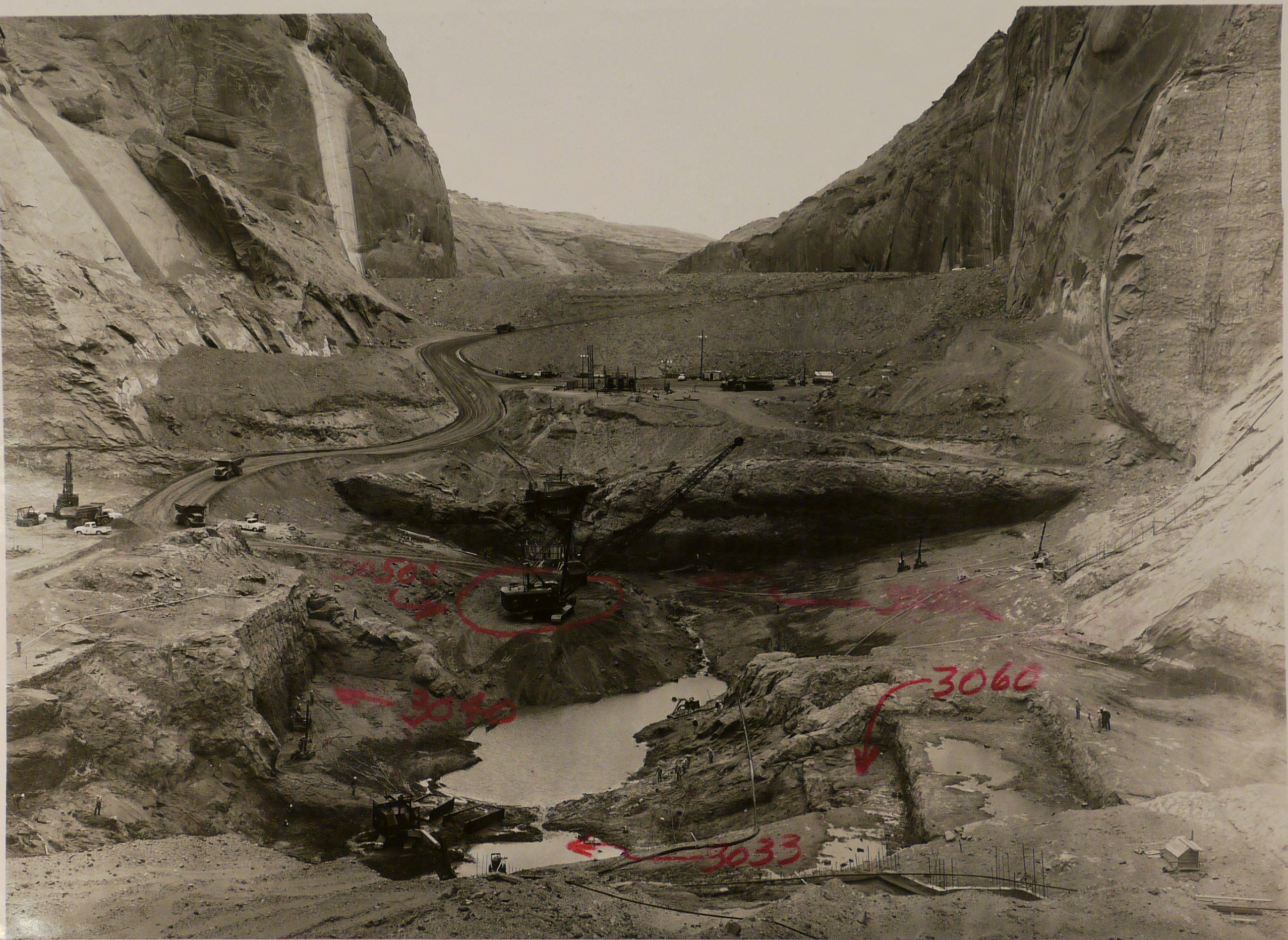
557-420-04764 Glen Canyon Unit--C.R.S.P. Looking upstream at excavation in the river bottom for power plant and dam foundation. Contractor: Merritt-Chapman and Scott Corporation, Contract No. 14-06-D-2403, Specs. No. DC-4825. 4-28-60 A. E. Turner
