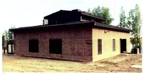
Pump station would be designed to withdraw 250 million gallons of water per day using eight pumps and eight natural-gas driven engines. Note: building dimensions would be approximately 140 feet x 170 feet with a height of 40 feet.
