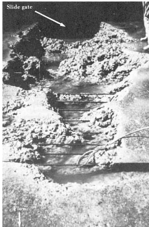
FIGURE 3-17.—Palisades Dam, outlet works vortex caused damage downstream of slide gate.
