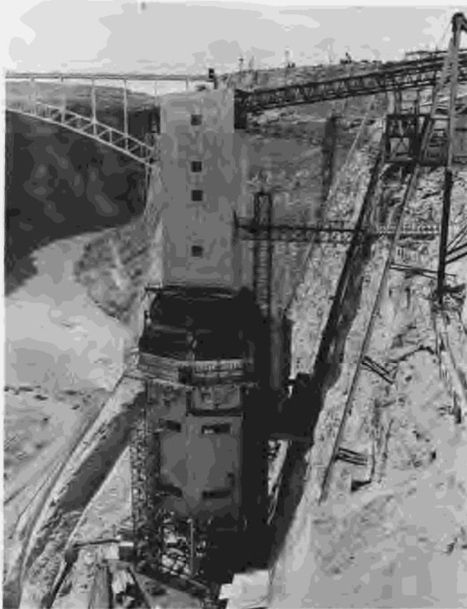
Figure 246.—Concrete batching plant being set up on west rim of Glen Canyon. P557-420-4781, April 29, 1960.
