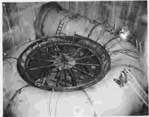
Figure 286.—Powerplant distributor tube for unit bay 2 being welded. P557-420-8176, April 11, 1963.
