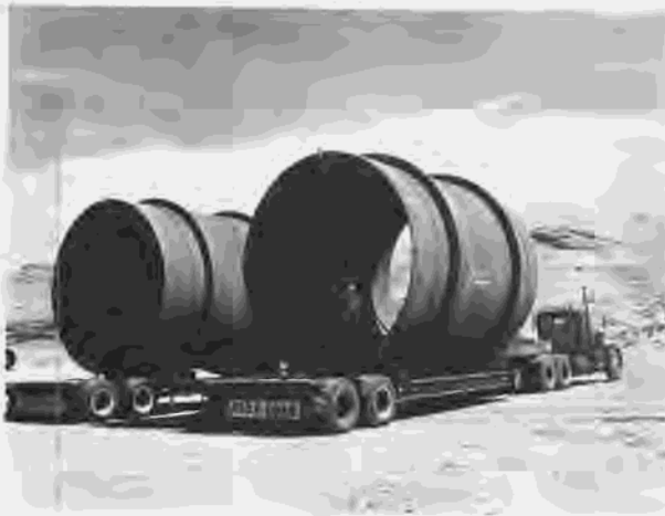
Figure 272.—First of the penstock sections arriving at the damsite. These penstock sections are 15 feet in diameter and 20 feet long. The sections were shipped by rail from California to Flagstaff, Ariz., and trucked to the damsite. P557-420-5052, July 9, 1960.
