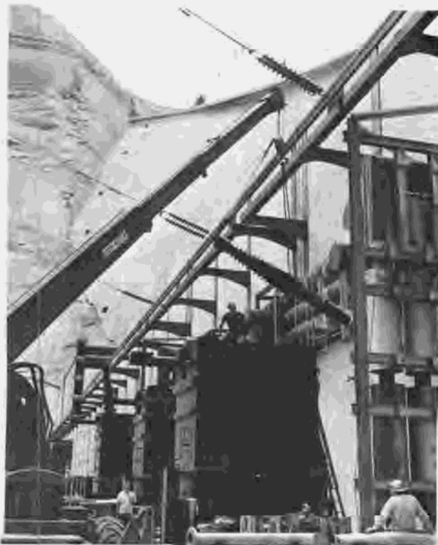
Figure 291.—High-tension bushing being raised into place on transformer K7A. P557-420-9847, June 10, 1964.
