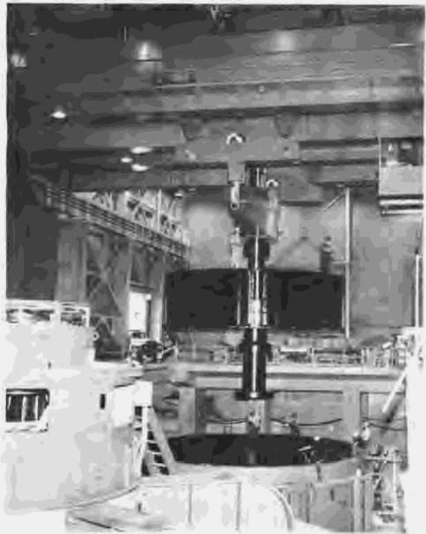
Figure 288.—Rotor for generating unit 8 being lowered into stator. P557-420-11335, July 21, 1965.
