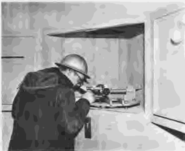
Figure 267.—Plumbine well reading station in block 4 of dam at elevation 3390.00. P557-420-9334, February 7, 1964.
