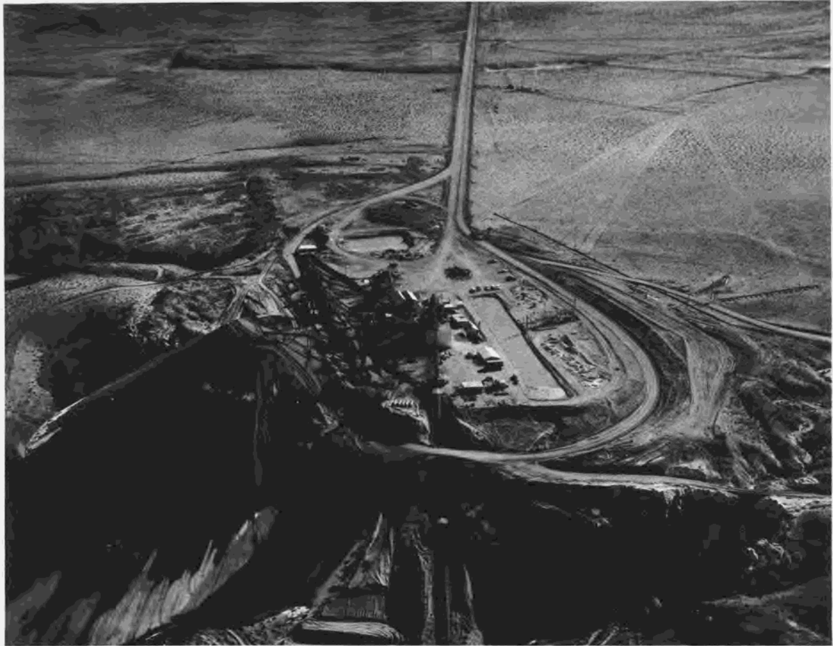
Figure 245.—Aerial view of aggregate processing plant on ledge above Wahweap Creek. P557-420-5568, December 14, 1960.
