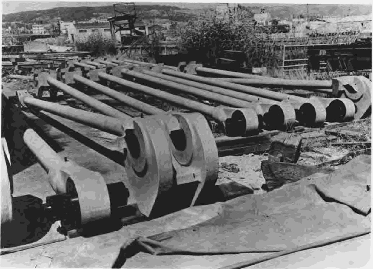
Figure 147.—Intermediate stems and coupling hooks for the 13.96- by 22.45-foot fixed-wheel gate. P557-D-37604.
