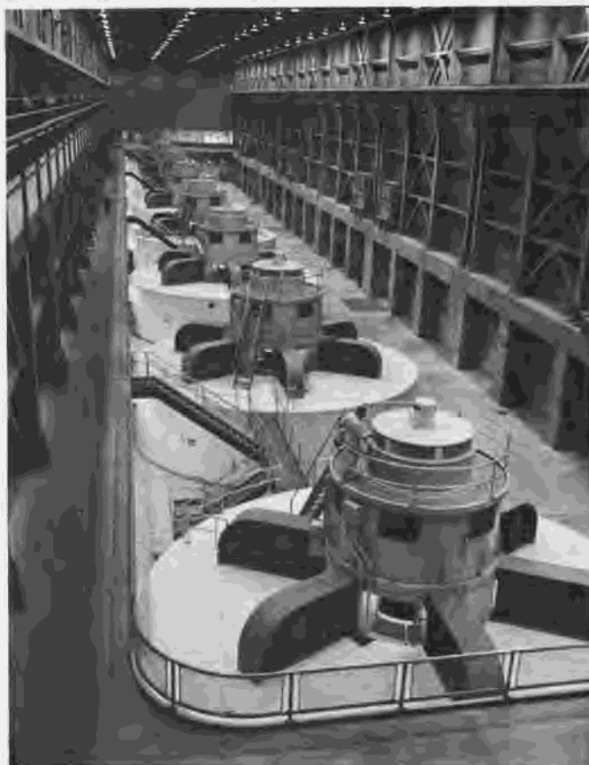
Figure 287.—Interior view of powerplant. The eight generating units have a total installed capacity of 900,000 kilowatts. P557-420-12678A, September 22, 1966.
