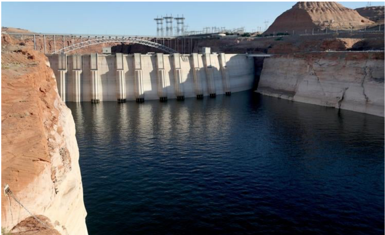
The exposed penstocks (intakes to the power turbines) on Glen Canyon Dam in the Glen Canyon National Recreation Area, Page, Ariz. The water level is at its lowest since 1967, when the dam was still being initially filled. Kelly Presnell Arizona Daily Star.
