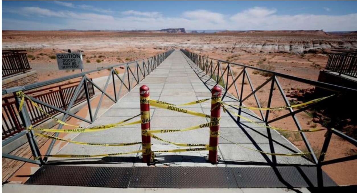
The entrance to the pedestrian access ramp of the Antelope Point Marina is taped off after being cutoff from the docks due to receding waters of Lake Powell. Kelly Presnell Arizona Daily Star.
