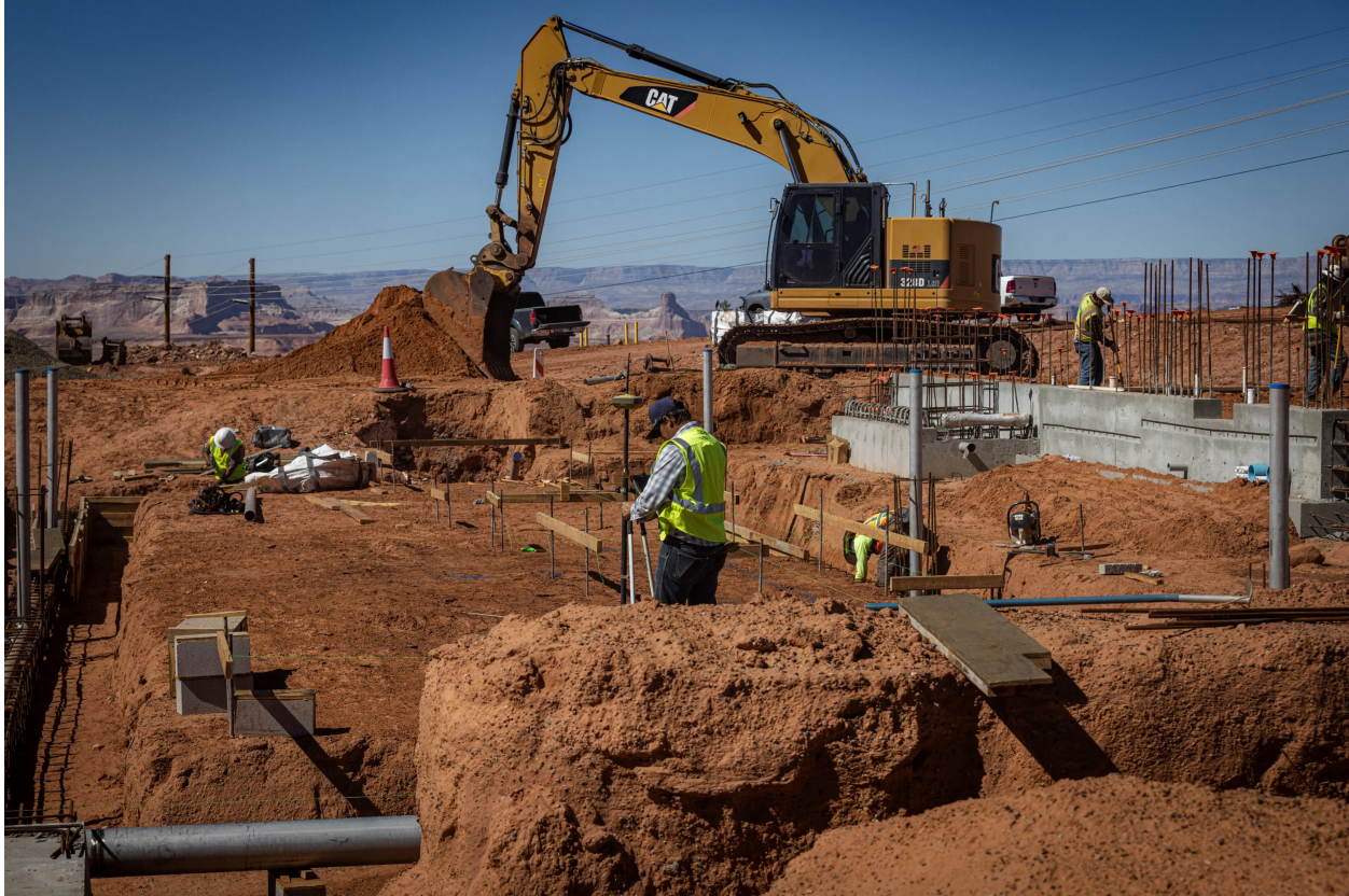
Photo caption: A construction crew installs pipes at the new LeChee Water Treatment Plant near Lake Powell, along the Arizona-Utah border. Sharon Chischilly for ProPublica.
