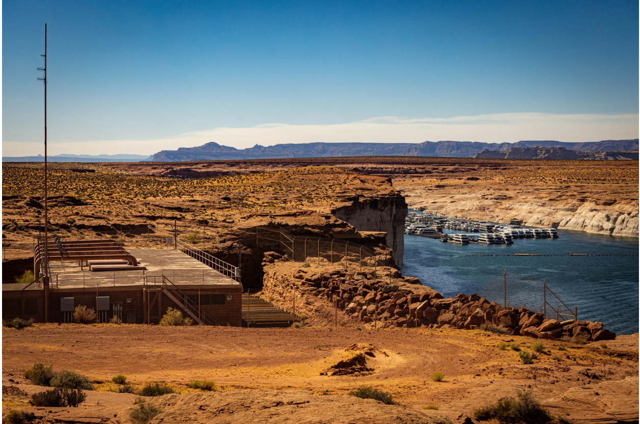
Photo caption: The former Navajo Generating Station's intakes, which drew water from Lake Powell to cool the coal power plant, sit unused, awaiting funding from the stalled settlement. Sharon Chischilly for ProPublica.
