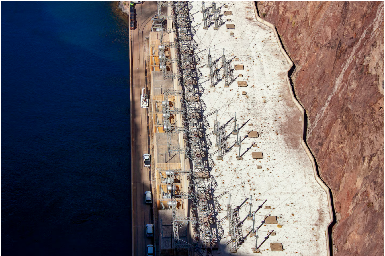
(Brett Walton | Circle of Blue) Morning sun strikes the powerhouse on the Nevada side of Hoover Dam.
