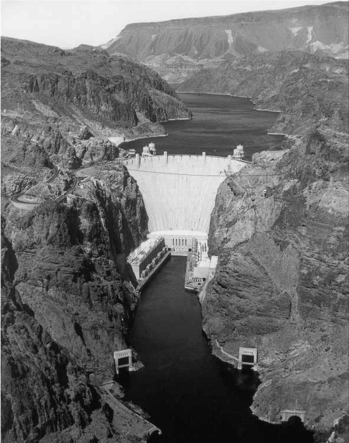
Figure 12 - Hoover Dam: Downstream face showing powerhouses. Source: Bureau of Reclamation.
