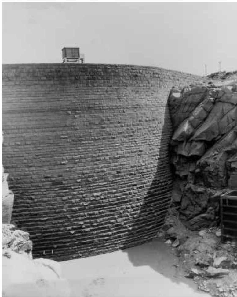
Figure 5 - Pathfinder Dam on the North Platt River near Casper, Wyoming is a masonry arch and cantilever section . Source: Bureau of Reclamation
