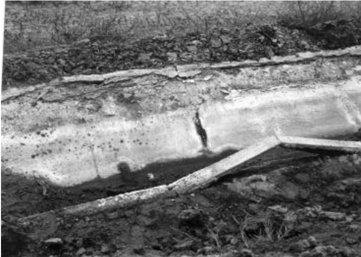
Figure 1 Sulfate attack on a five year old concrete canal lining, Central Valley Project, California. The groundwater sulfates infiltrate the concrete and chemically react with certain cement hydration products. The expansive reaction causes cracking and disintegration of the cement paste matrix. Notice the deterioration near the upper soil strata where the sulfates are more concentrated.
