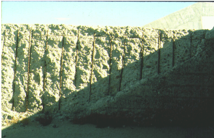
Figure 3 Freezing and thawing deterioration of a spillway training wall at Lahontan Dam in California. The “sand cement” concrete placed in 1915 was severely damaged by freezing and thawing in the colder and mountain regions of the west. Notice the shady area is less damaged than the section exposed repeatedly to cold temperatures followed by the
