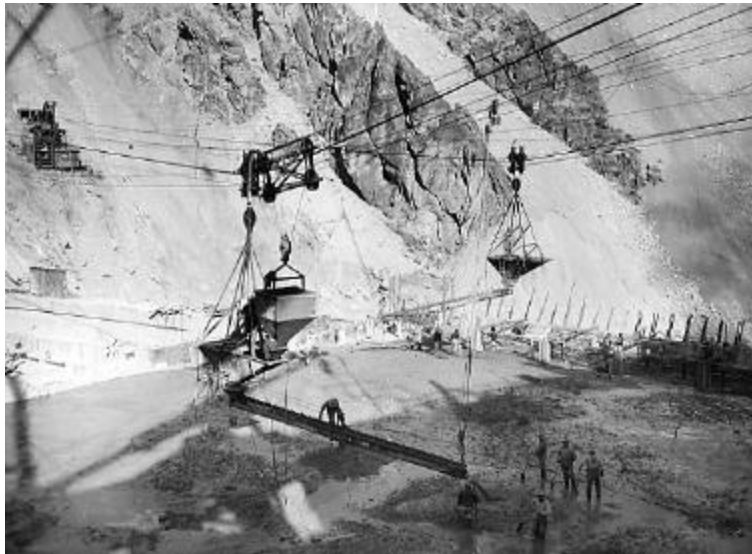
Figure 4 Chuting wet concrete into place - Arrowrock Dam, about 1912. Elaborate chute systems required a very fluid concrete mixture to be placed and spread in the forms. Water was the “admixture” of choice to improve the fluidity! Bureau of Reclamation Historical Photographs.
