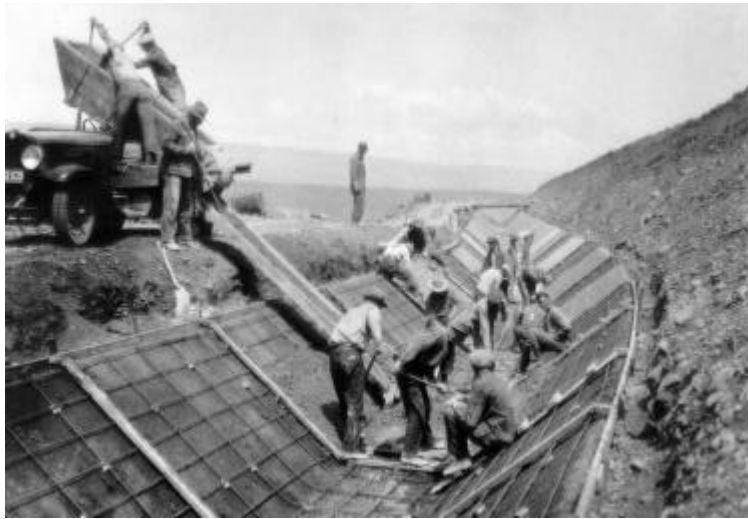
Figure 5 Early concrete canal lining. Horse and buggy transporting gave way to central batch plants and the first motorized transporting buggies. Still the concrete placing and compacting processes were performed by laborers with shovels. Bureau of Reclamation Historical Photographs.
