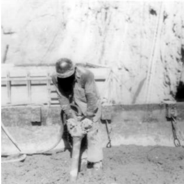
Figure 7 The mechanical concrete vibrator was first introduced to the Bureau of Reclamation during construction of Hoover Dam. The laborers job of hand-tamping and spading was replaced with mechanical equipment. However, even though the consolidation process was accomplished by machine, it took a strong person to manipulate these vibrators! Bureau of Reclamation Historical Photographs.
