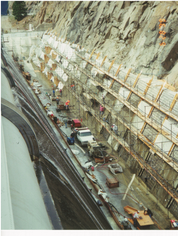
Figure 8 Tieton Dam spillway reconstruction, 1999. Yakima Project, Washington. The challenge for the 21 st Century. Identify, protect, and preserve. The spillway was completed in 1925 and suffered from severe freezing and thawing deterioration. The spillway was extensively repaired after about 40 years and reconstructed in 1999. These types of rehabilitation efforts will take center stage in 21 st Bureau of Reclamation construction. Construction Records, Yakima Construction Office, Washington.
