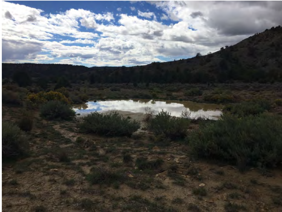
Figure 15: View facing east of a sediment pond just above PJD2a. The pond's basin was observed to be mostly full of sediment and does not appear to be currently functional. No wetland indicators were observed here.
