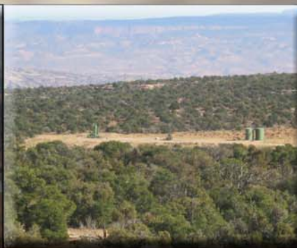
Oil and Gas Well in the Big Flat Area
