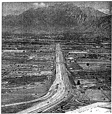
Ames was the lead civil contractor in a JV team (Provo River Constructors) on the I-15 CORE project, Utah's first "fixed price/best design" project delivery method. The massive rebuild of a 24-mile section of Interstate I-15 added two lanes in both directions and replaced or restored 63 bridges; the entire project was designed and built in less than three years.
