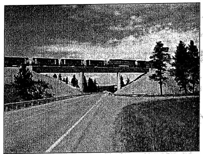
Ames Construction was the design-build general contractor for this 36-mile long railroad spur that included construction of five bridges. Under a very aggressive schedule, Ames crews moved 9.6 million cubic yards of earthwork in 9 months.
