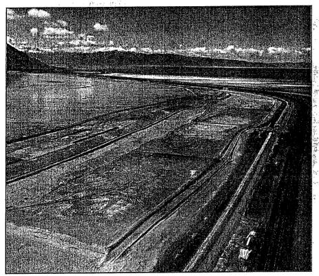
The Kennecott Utah Copper North Tailings Dam project represents a major expansion that is adding more than seven miles to an existing tailings dam. Kennecott generates mill tailings from its copper/molybdenum concentrator, and transports these tailings in slurry form via a 17-mile long pipeline to the North Tailings Dam.
