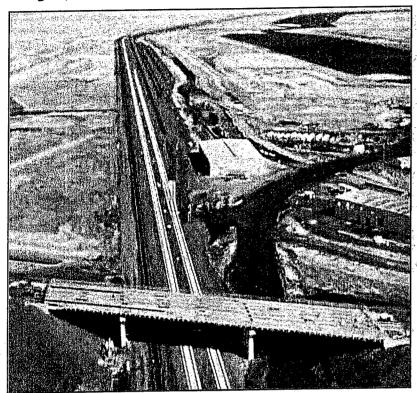
Ames Construction relocated 26 miles of mainline, spur and siding track for the Union Pacific Railroad to accommodate modifications to Kennecott Utah Copper's tailings impoundment facilities near Salt Lake City, Utah.
