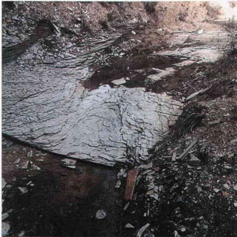
Photo 14 Klondike Canyon Seep - 03
