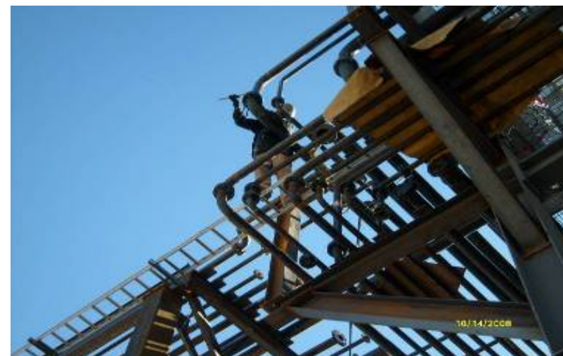
[ Pipe Line Connection on the Pipe Rack of Extraction Module ]
