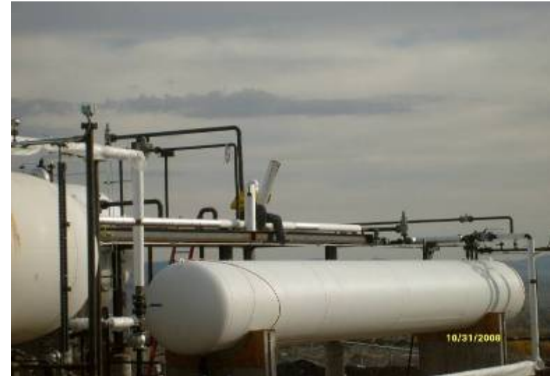
[ Insulation of New Pipe Lines to Storage and Bullet Tanks ]
