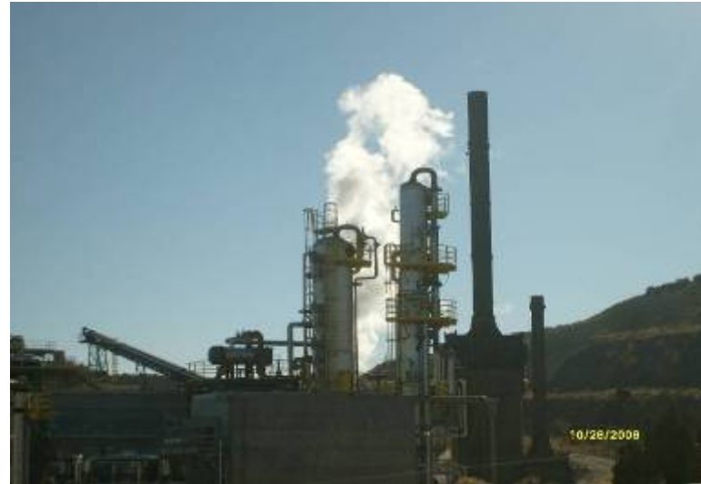
[ Pipe Line Steam Flushing from SRU to Flare ]
