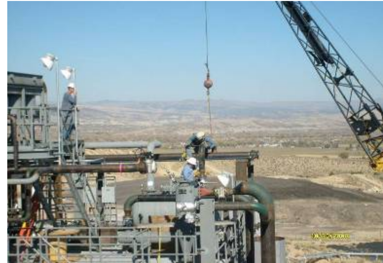
[ Pipe Line Connection of V-401 Vapor Line ]
