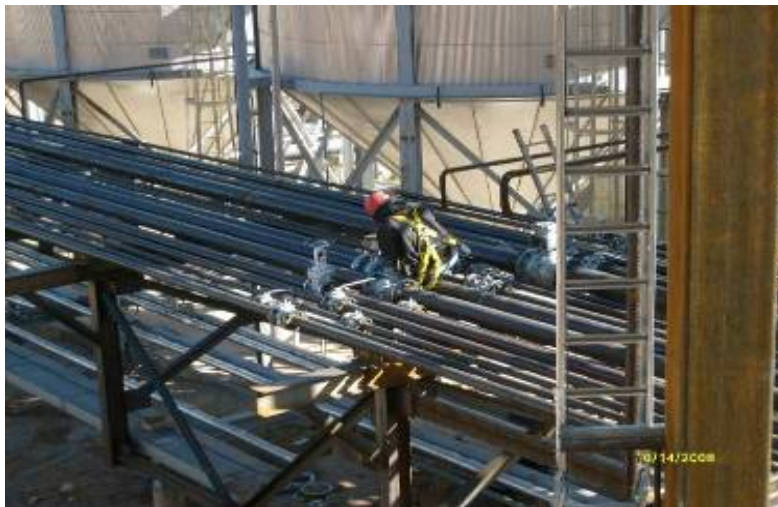
[ Pipe Line Connection on the Pipe Rack of Extraction Module ]
