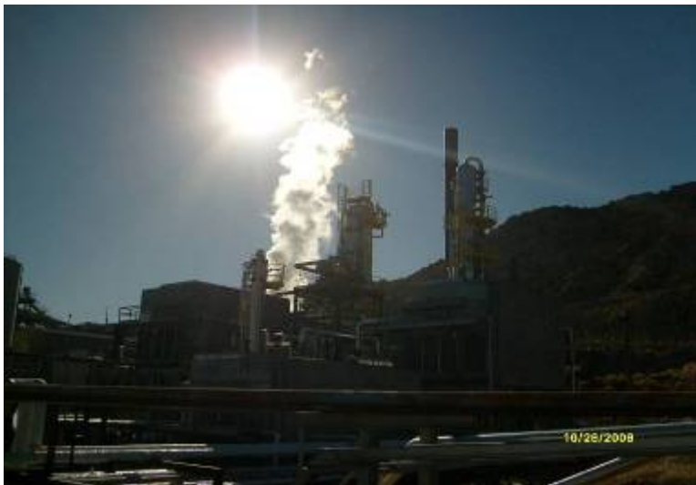
[ Pipe Line Steam Flushing from SRU to Flare ]
