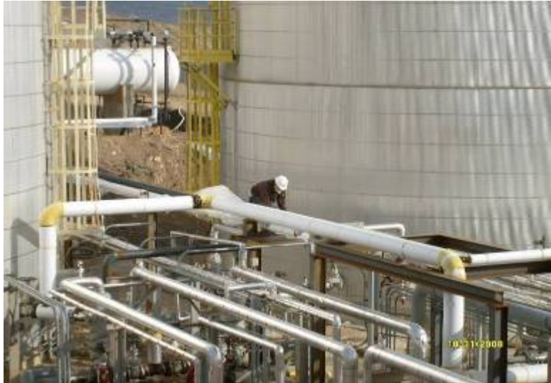
[ Insulation of New Pipe Lines to Storage and Bullet Tanks ]
