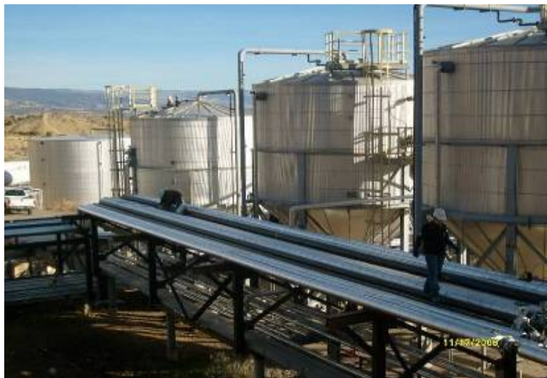
[ Insulation of New Pipe Lines to Storage and Bullet Tanks ]
